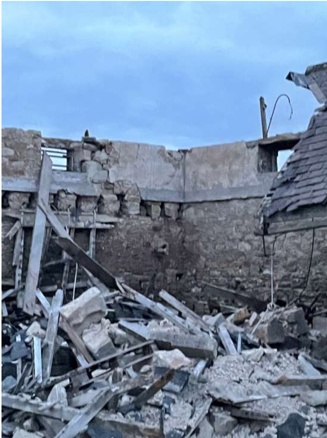
Interior NE corner of Building 1
