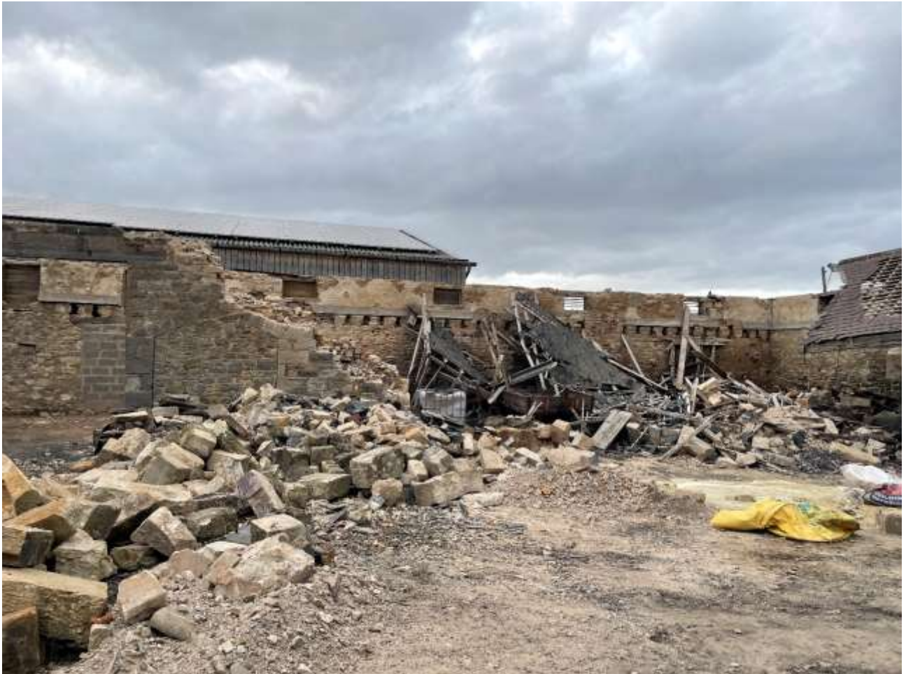
South elevation of the east half of Building 1
