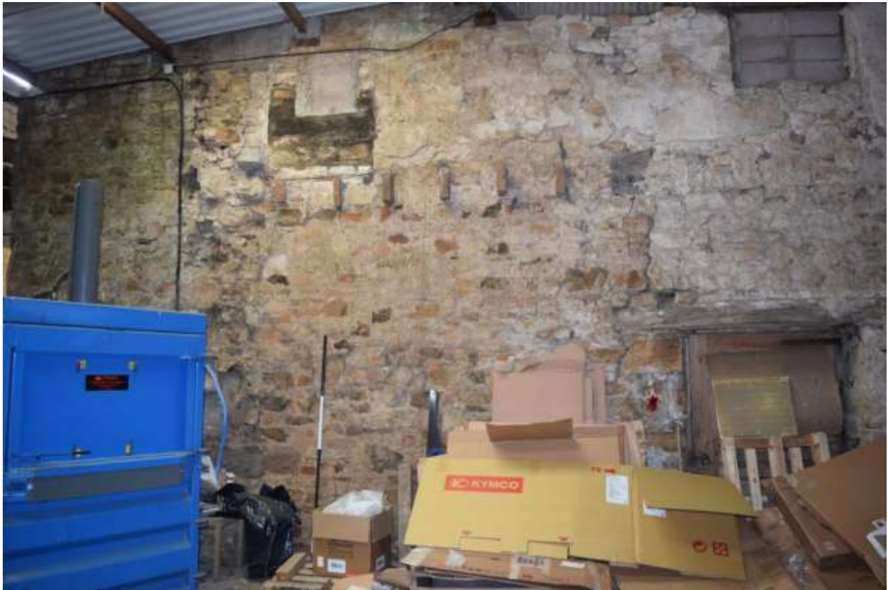
Detail of the remaining gable of Building 1 within Building 3
