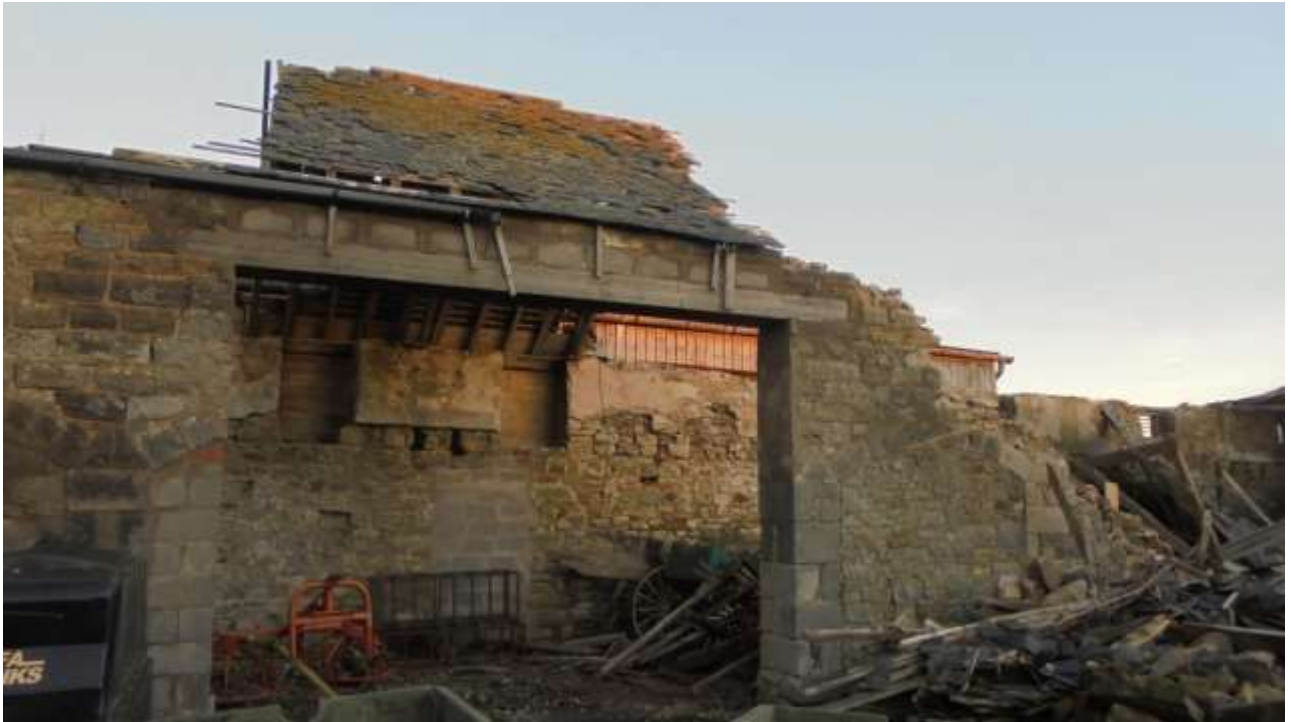
Detail of south elevation of Building 1
