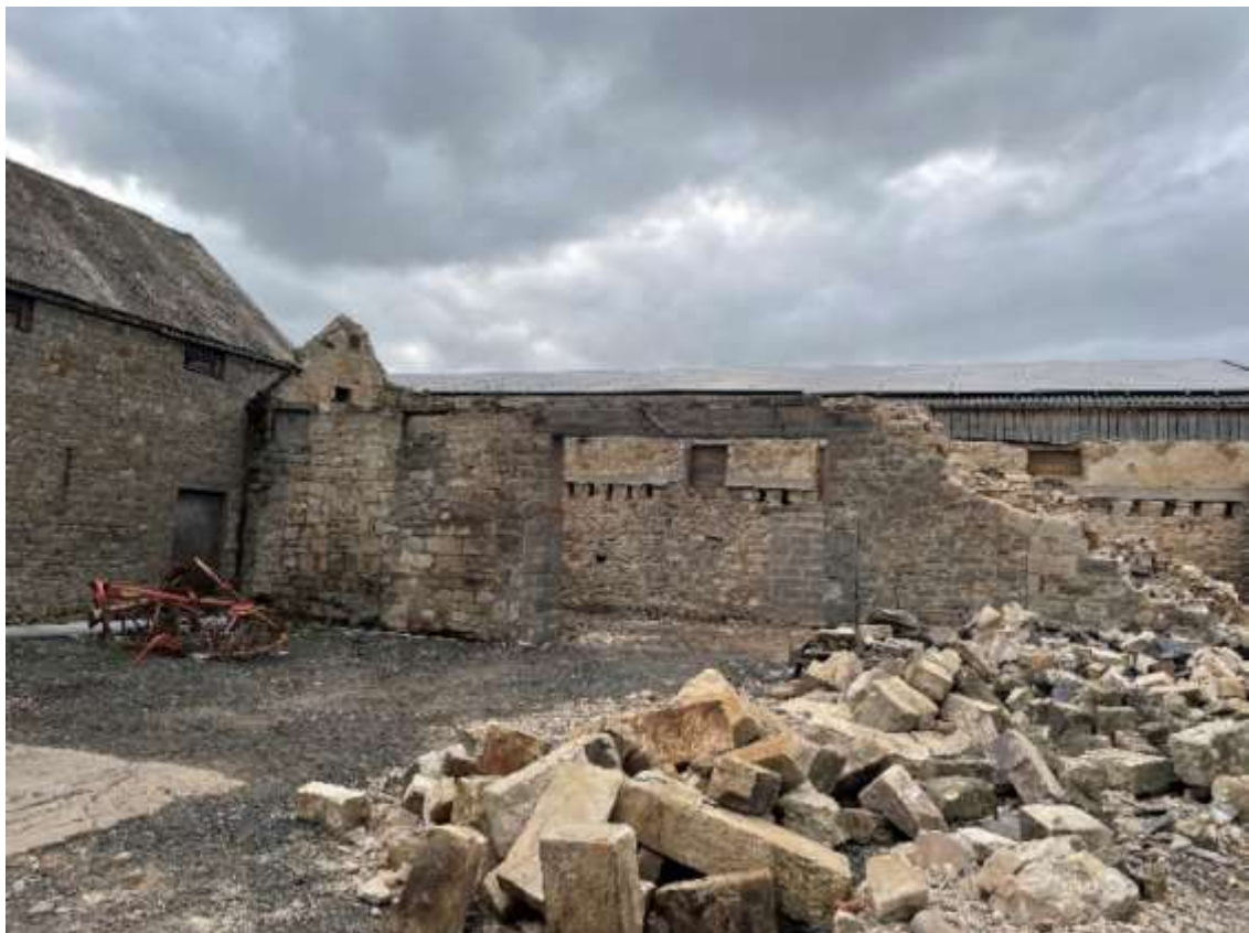
Figure 11. Detail of the south facing elevation of Building 1
