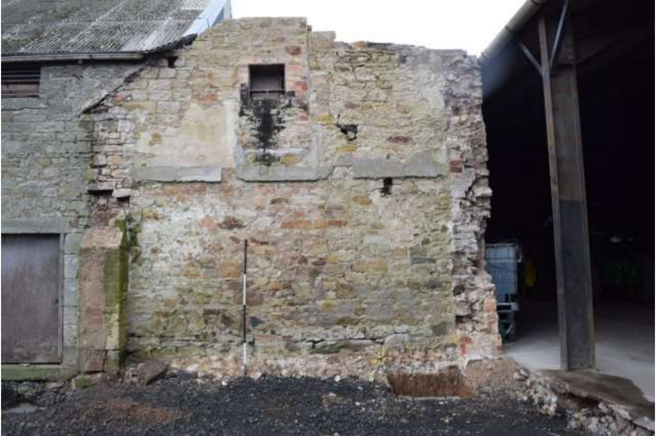
Detail of the remaining gable of Building 1
