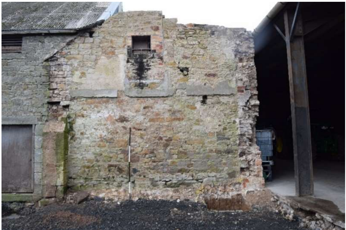
Figure 10. Detail of the internal east facing gable of Building 1
