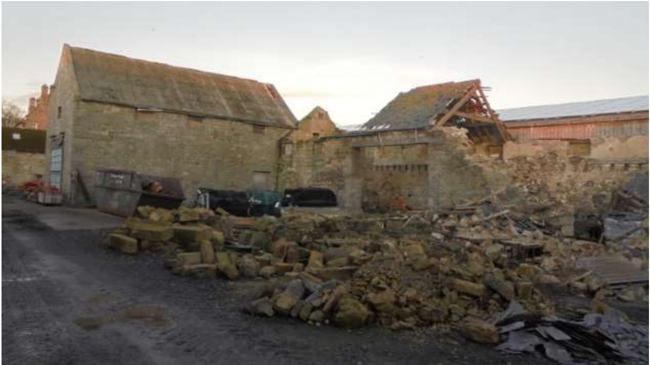
Remains of south elevation of Building 1
