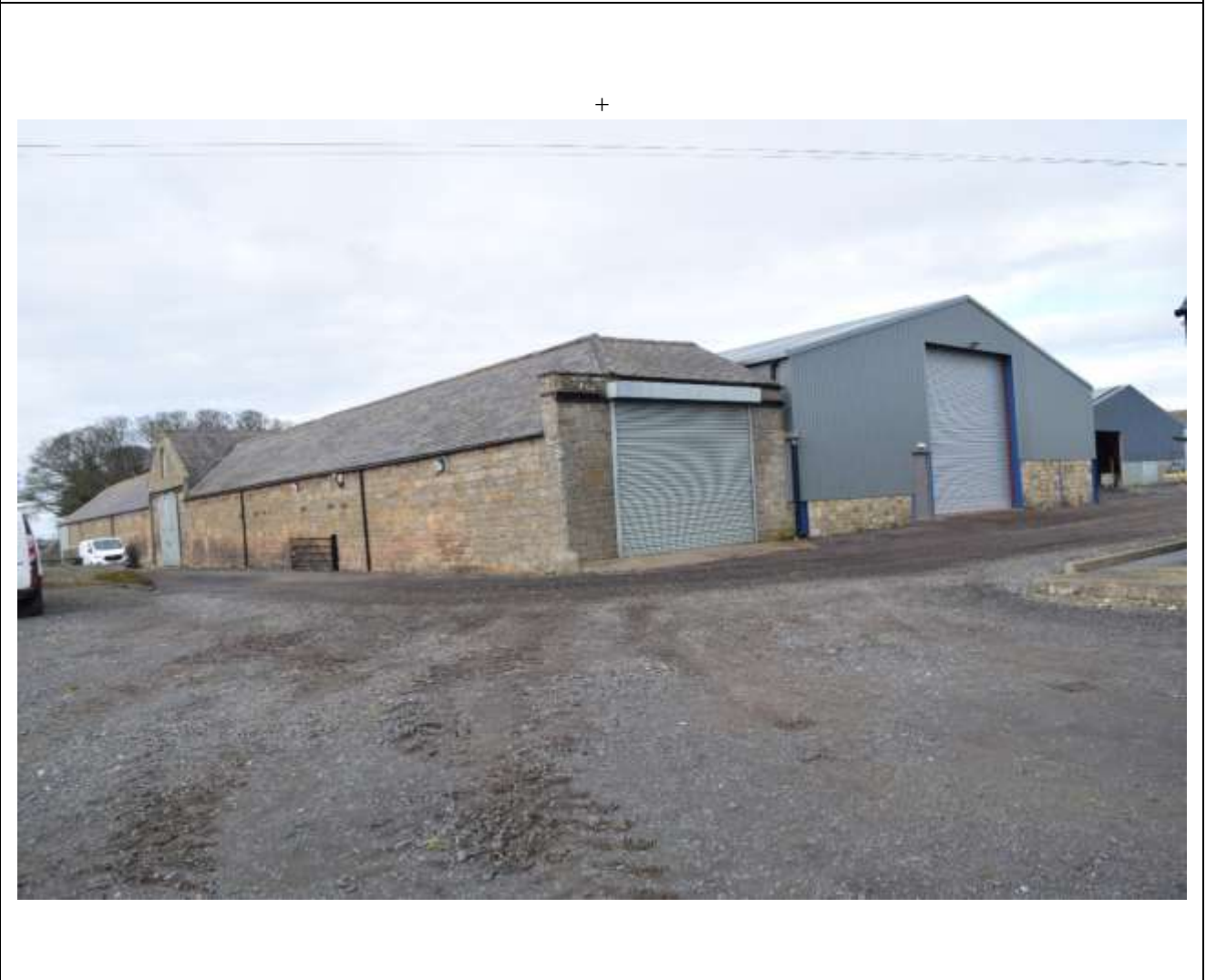
View of the south range including the original entrance
