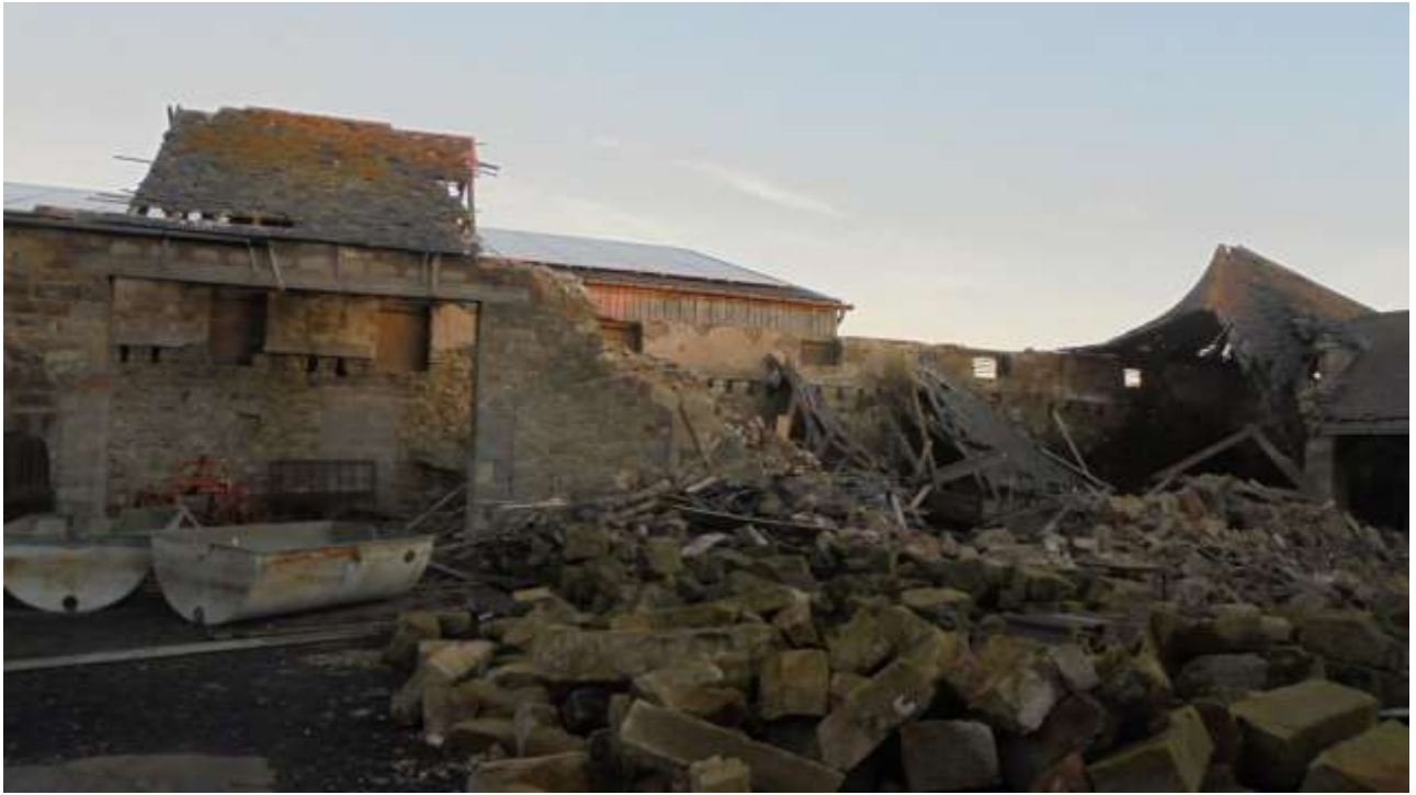
Remains of south elevation of Building 1
