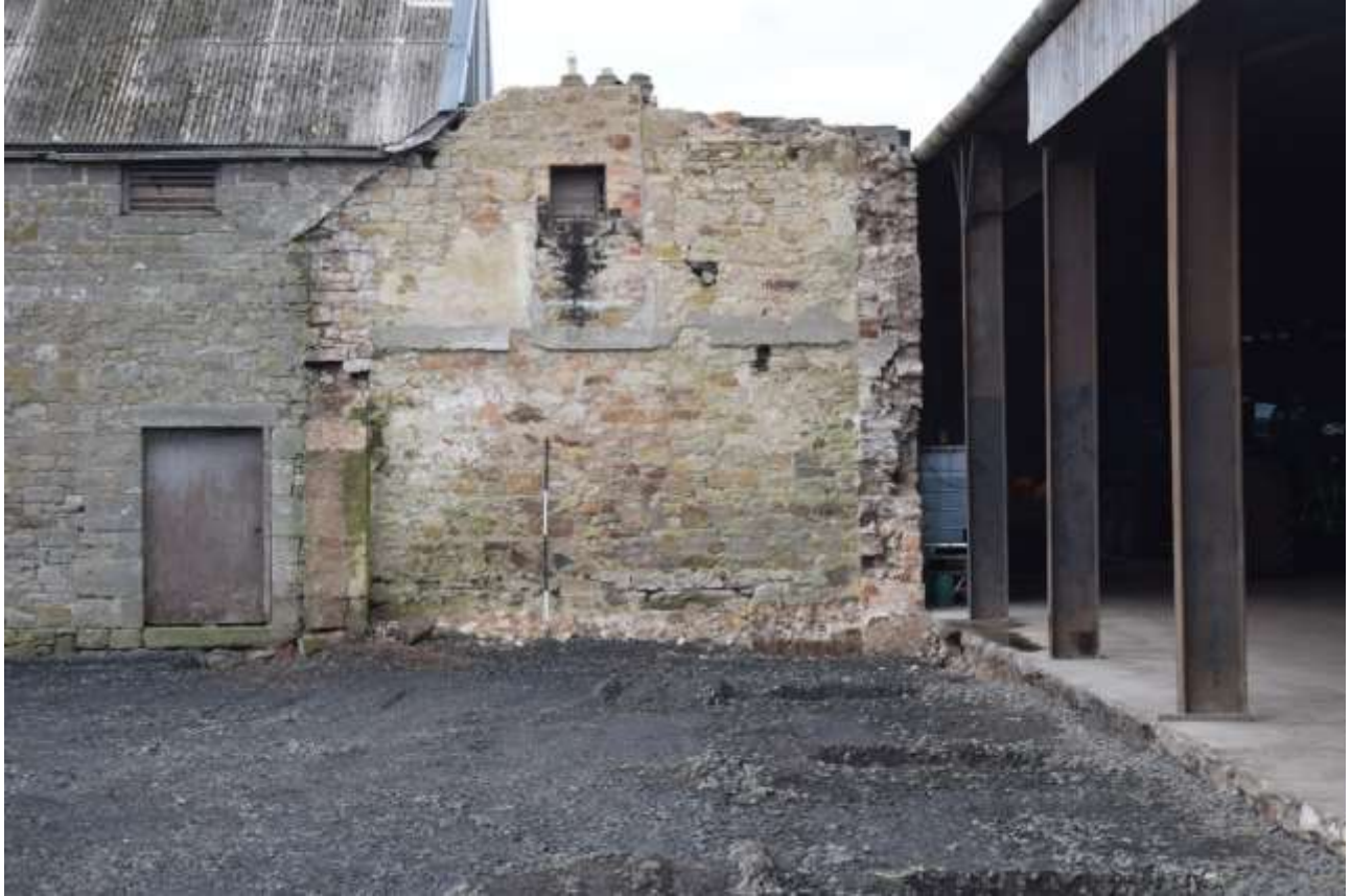
Detail of the remaining east facing gable of Building 1
