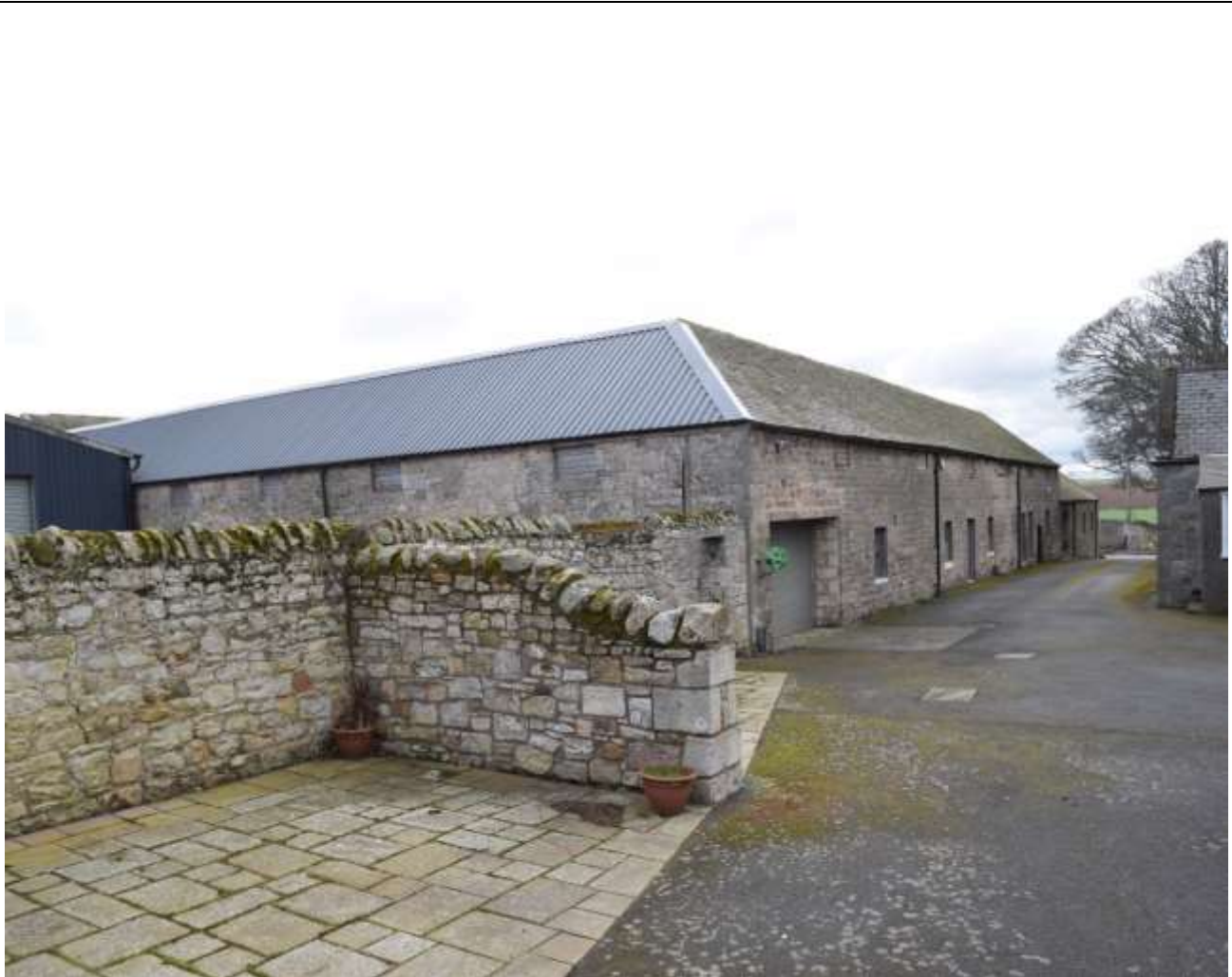
External west elevation of the west range, Building 5
