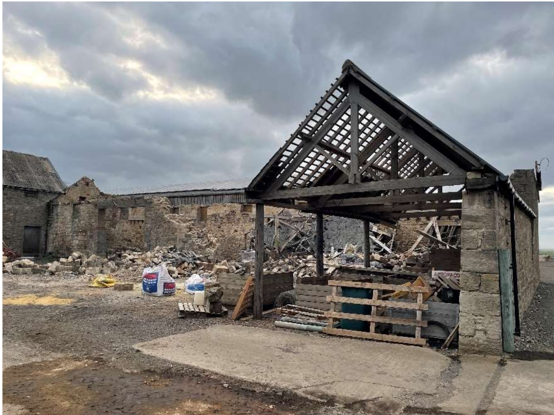
Figure 12. View of Building 2 facing north
