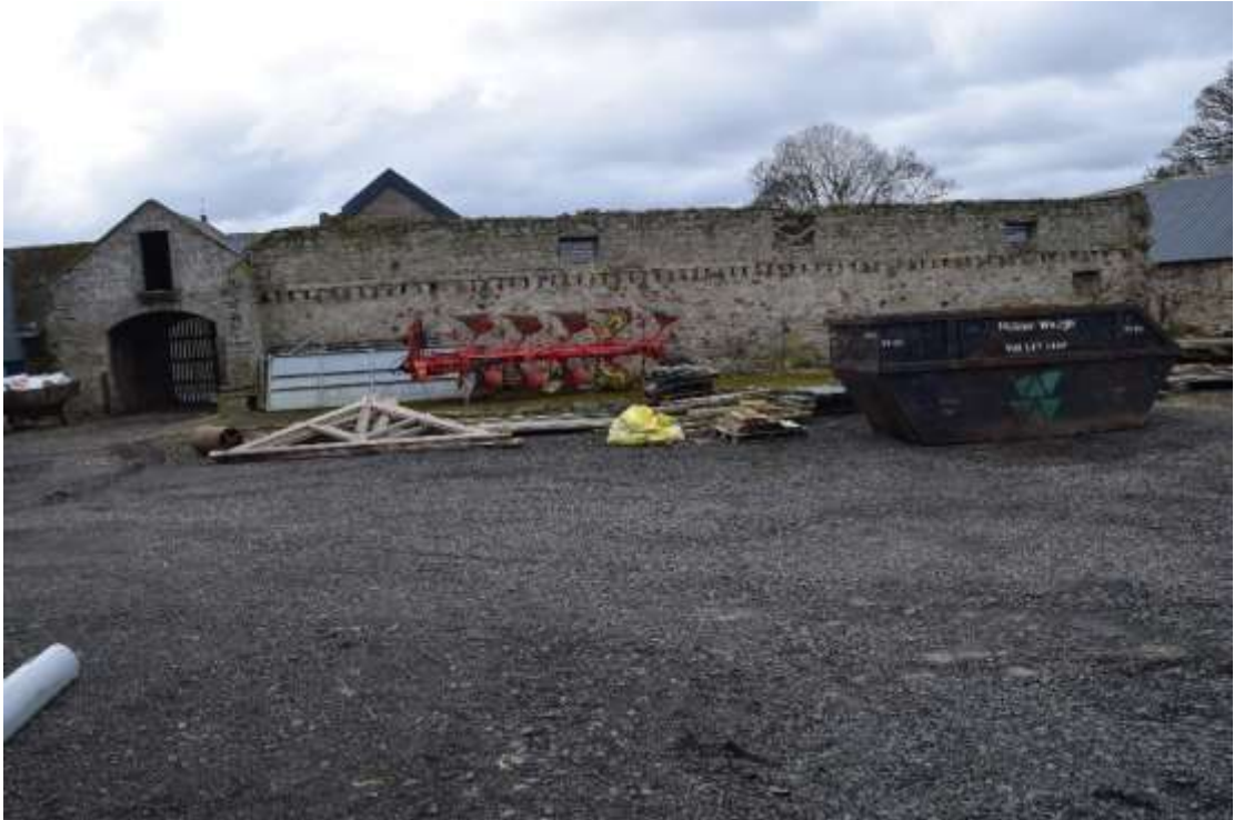
Figure 15. View of the surviving wall of Building 6 facing south
