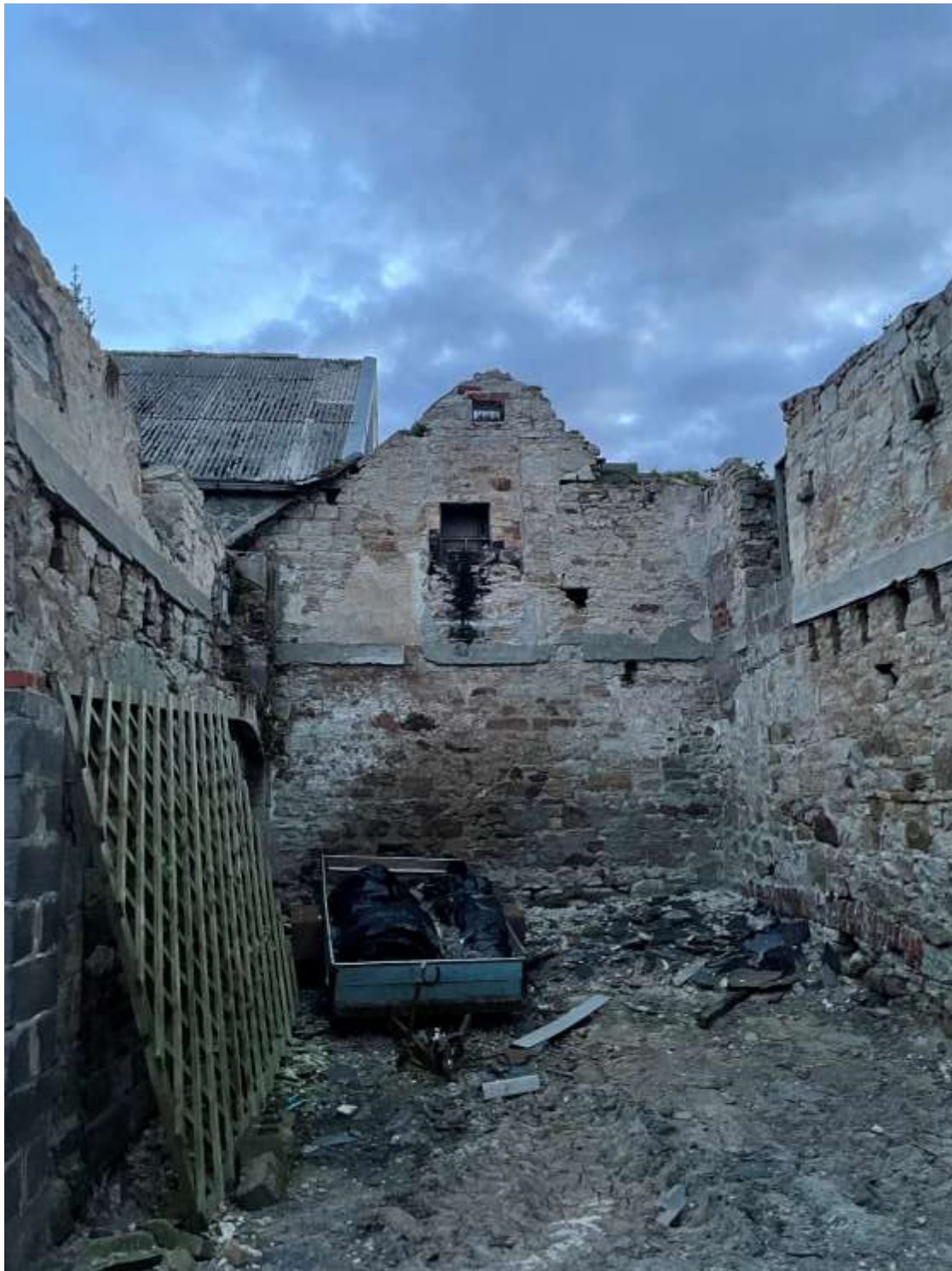
Interior view of west gable of Building 1
