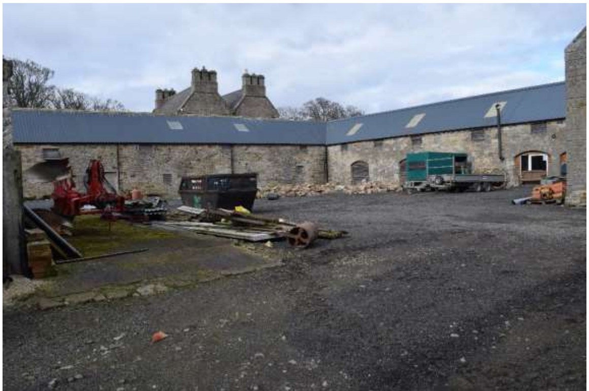
Figure 14. View of Buildings 4 and 5 facing north-west
