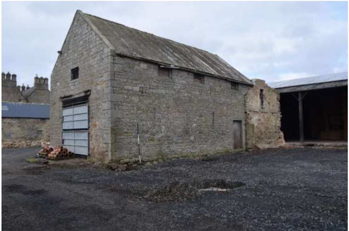
Figure 13. View of the south and east elevations of Building 3
