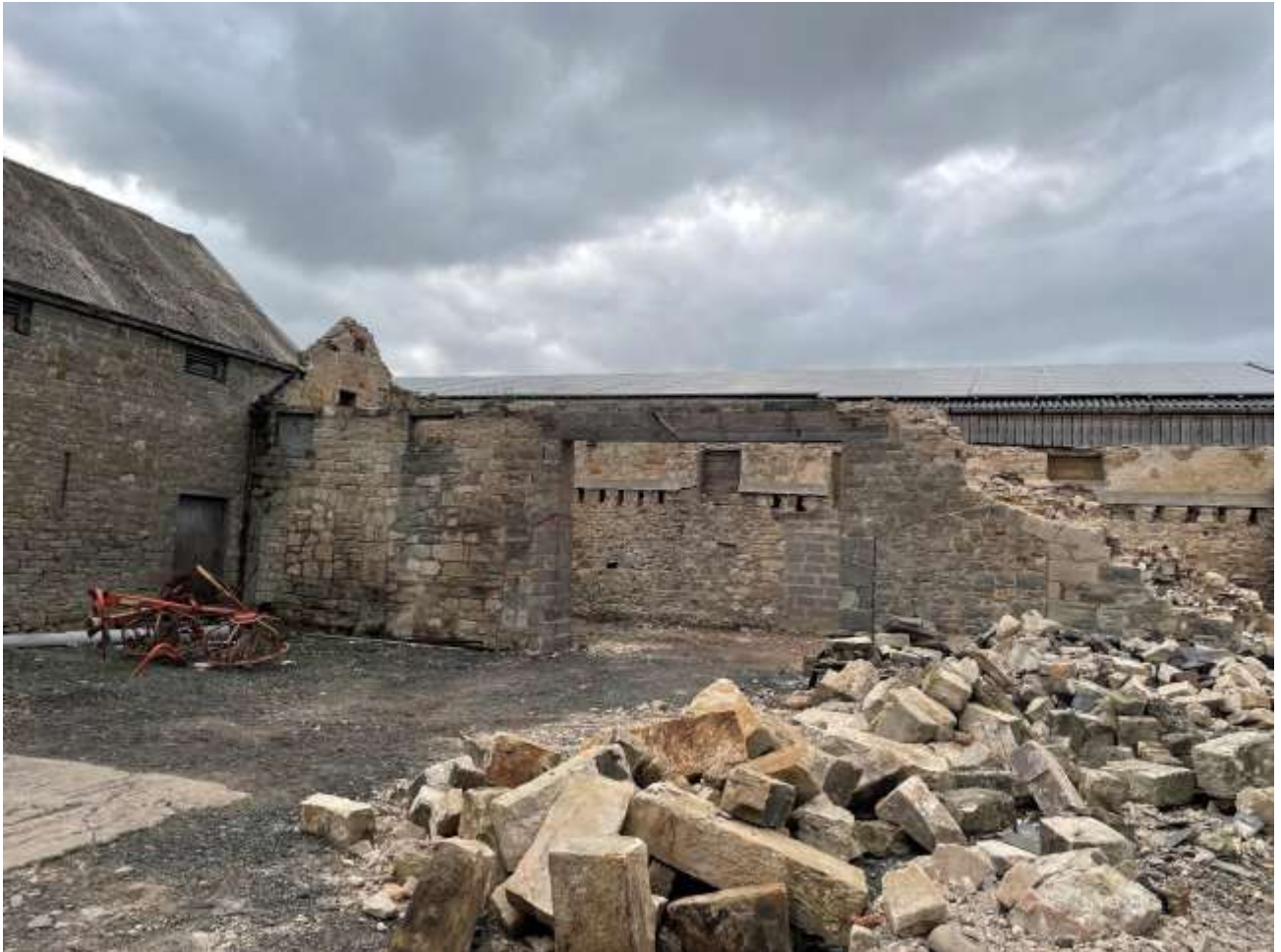
South elevation of the west half of Building 1
