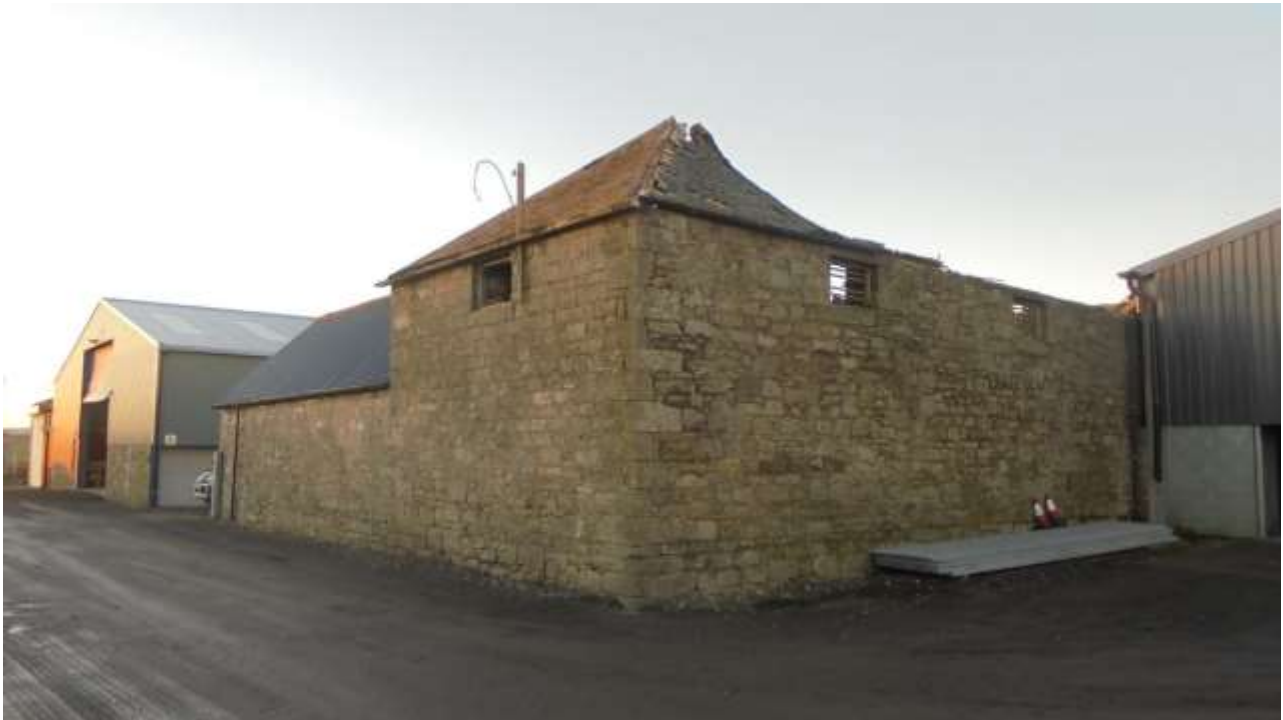
NE corner of Building 1 and 2
