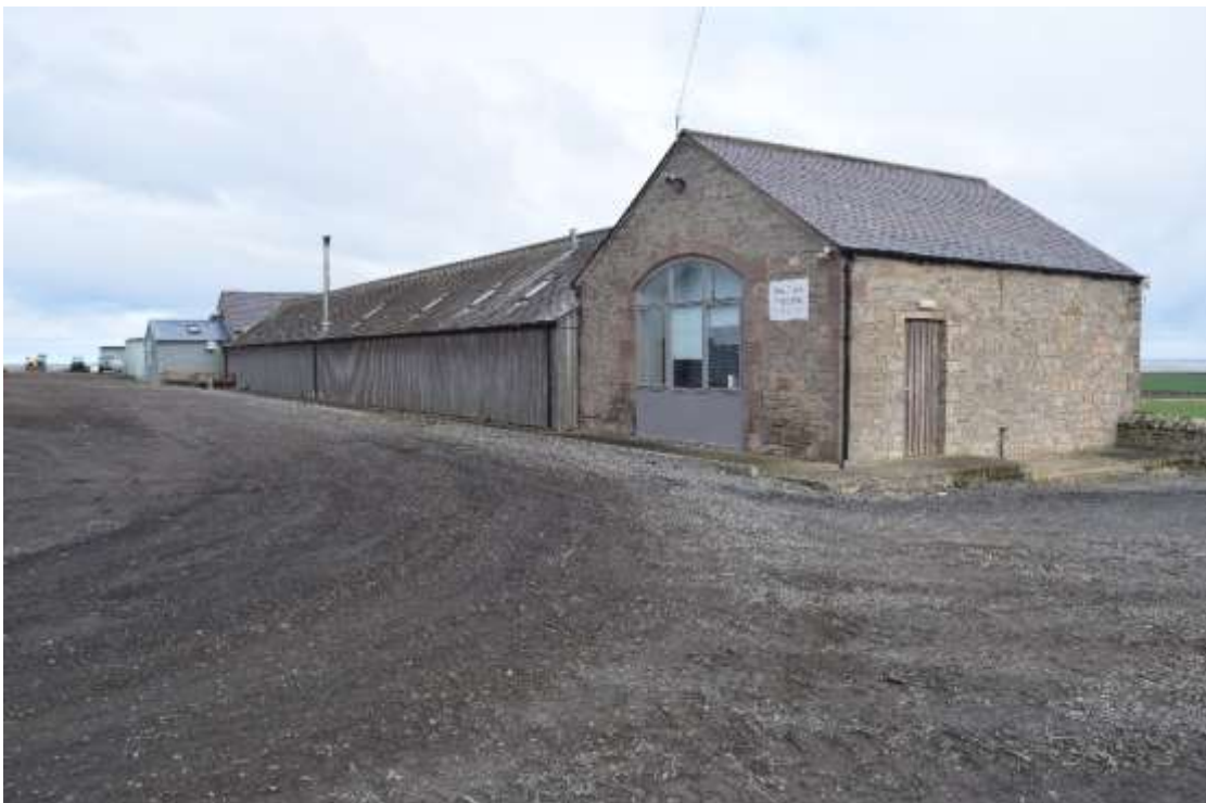
Figure 16. View of Buildings 8 showing the west and south walls, facing north-east
