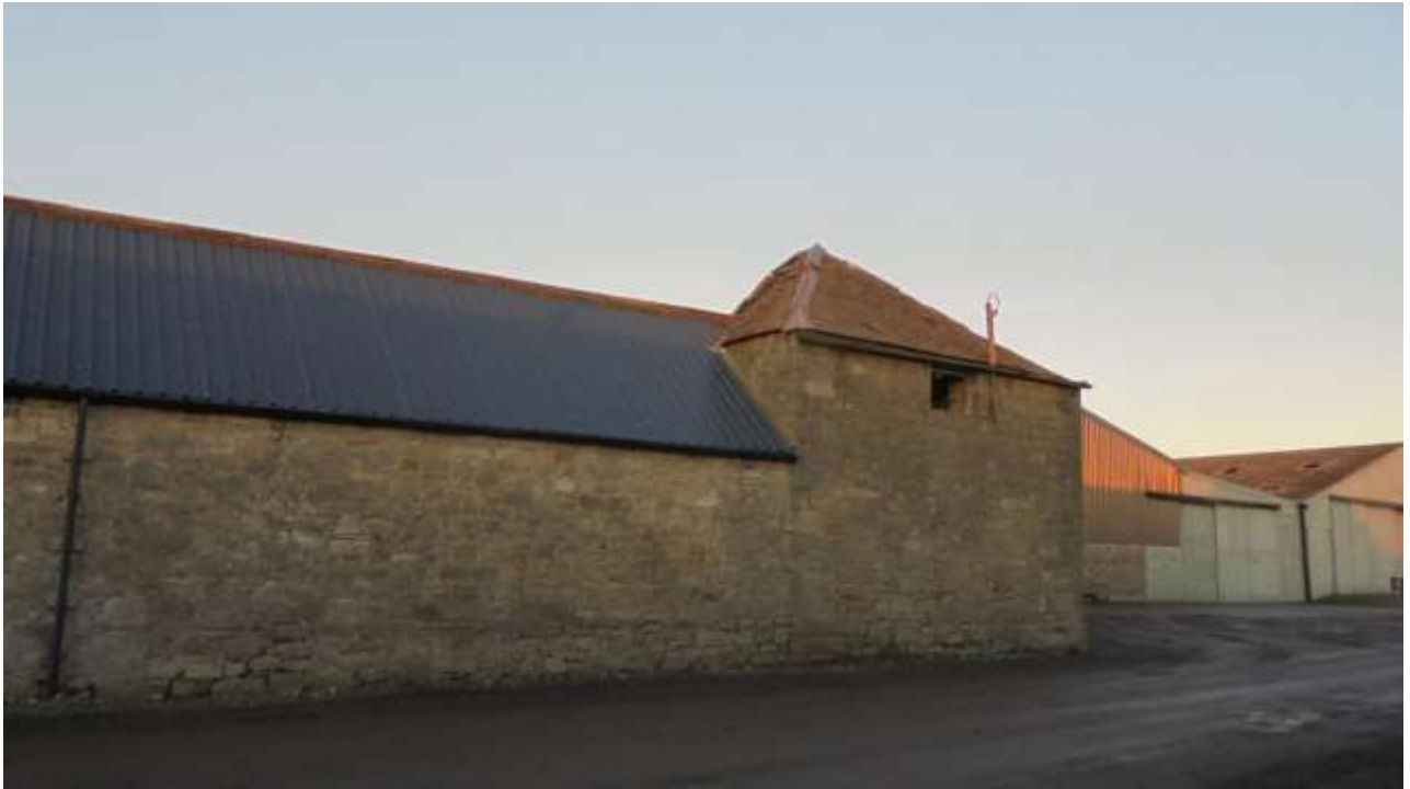
View of Building 2 and gable end of Building 1
