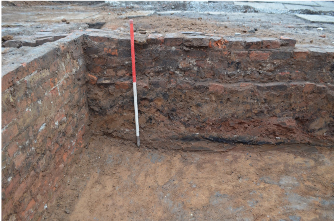
Illus 50. Phase 4 wall [38] constructed over in fill [40]. View looking south, scale 1 m.
