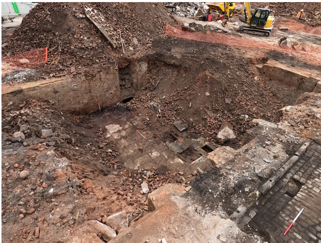
Illus 17. Overview of Phase 1 basements on eastern side of the site. View looking south-west, scales 1 m.
