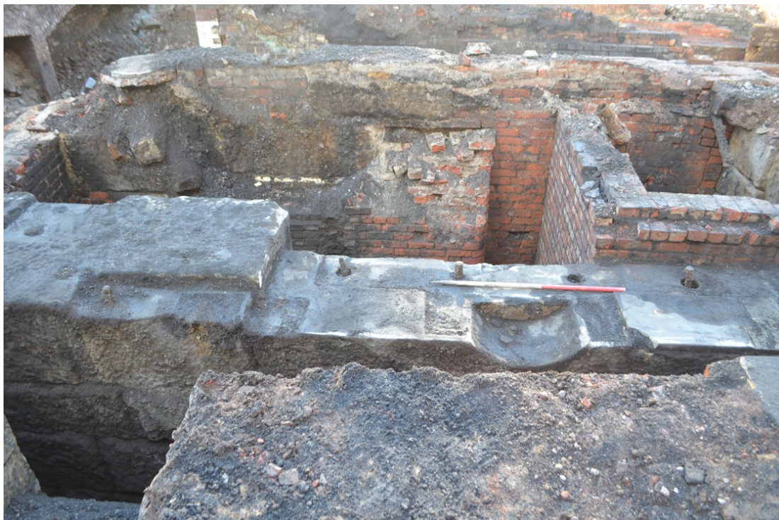
Illus 27. Detail of wall [94] in the Engine House showing the mounting for the flywheel and the possible second motion gear to the left. View looking east, scale 1 m.
