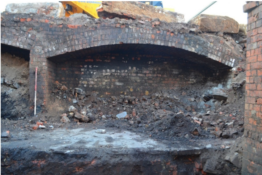
Illus 49. Storage recesses in wall [99]. View looking north, scale 1 m.
