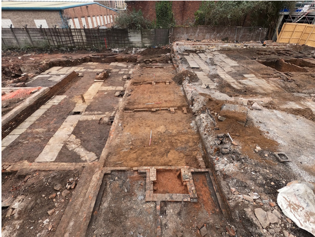
Illus 36. Overview of the Phase 2 blind back houses and factory extension. View looking west, scales 1 m.
