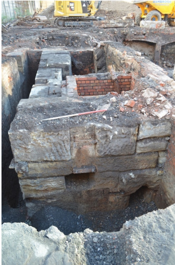
Illus 26. Detail of the central block carrying the mounting post for the beam. The openings in the masonry would have carried the pipework from the pump to the condenser tank in the foreground. View looking north, scale 1 m.
