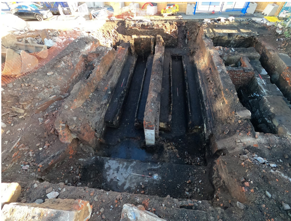
Illus 45. Overview of the Phase 3 Boiler House. View looking south, scales 1 m. The Phase 1 Engine House is on the right.
