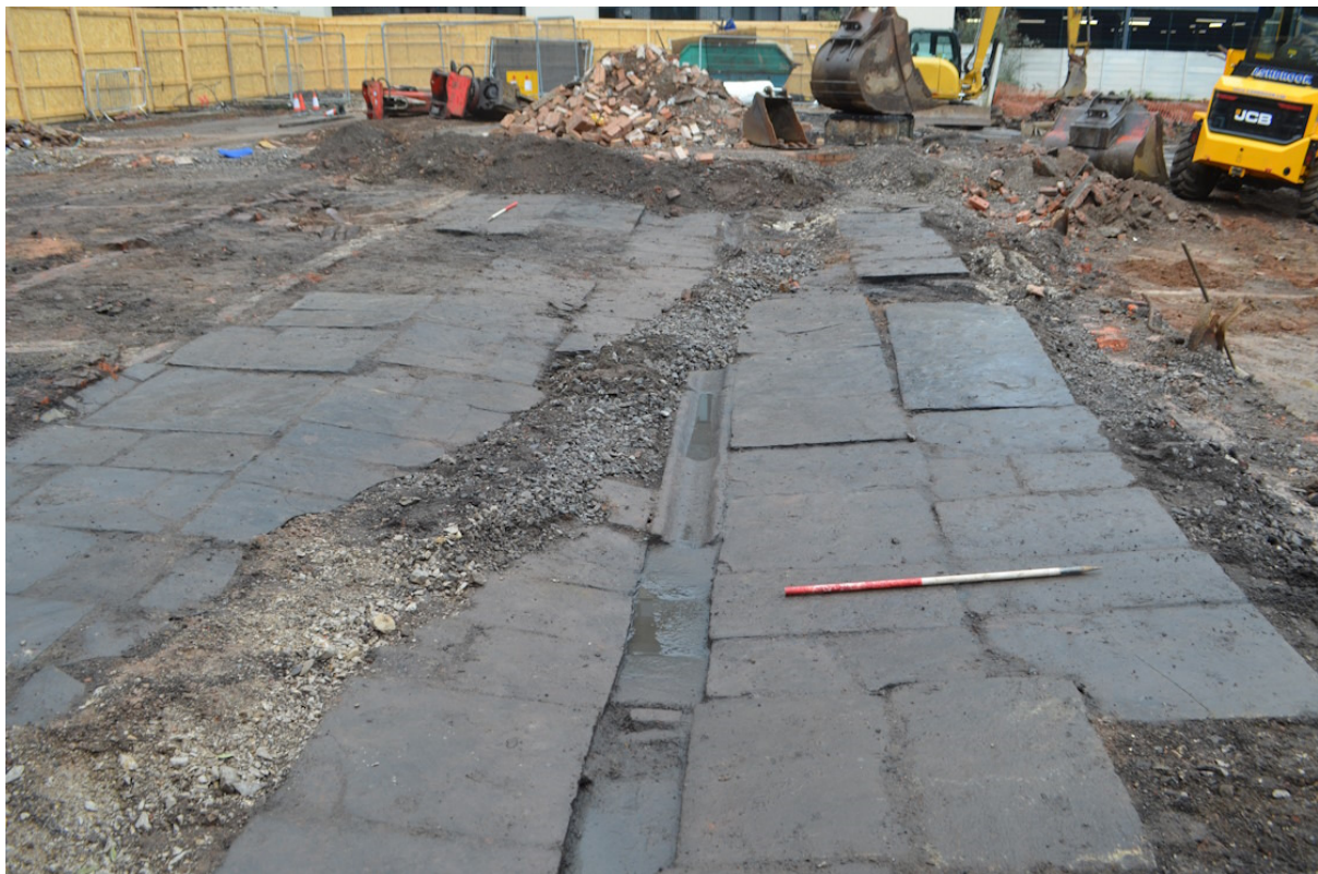
Illus 31. Flags surfacing Grey Place, note the drainage gully in the centre. View looking east, scale 1 m.
