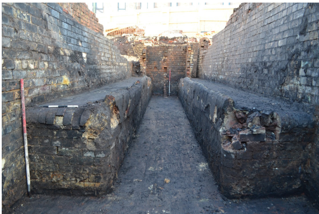
Illus 46. View along boiler bed [93] showing the mounting for the boiler. View looking south, scales 1 m.
