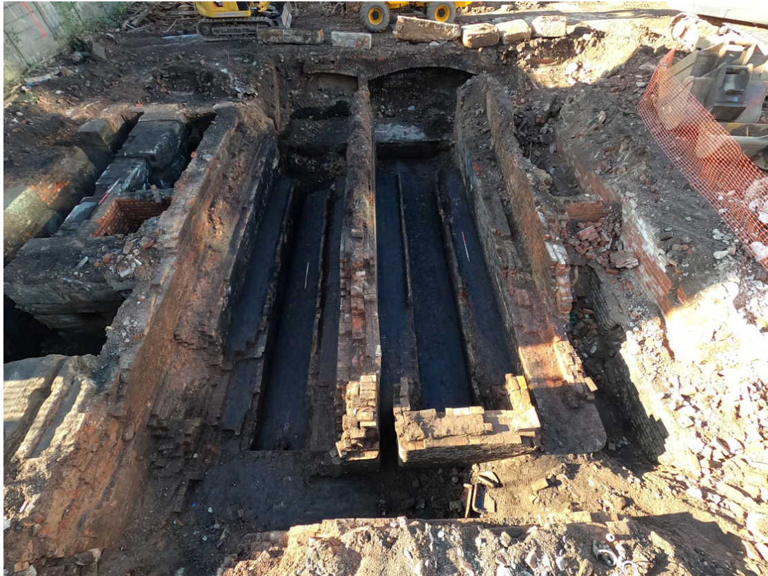
Illus 44. Overview of the Phase 3 Boiler House. View looking north, scales 1 m.
