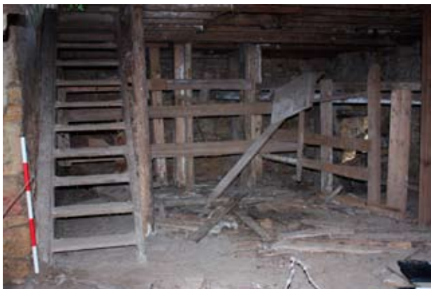
Illus 9 The ground floor stairs and wooden partition
