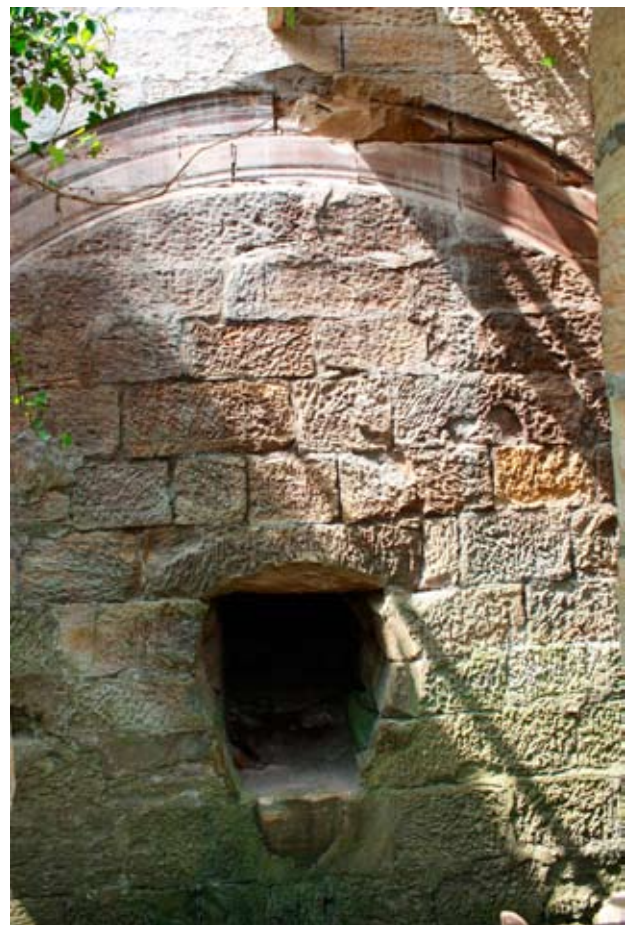
Illus 18 The axle aperture and water wheel grooves
