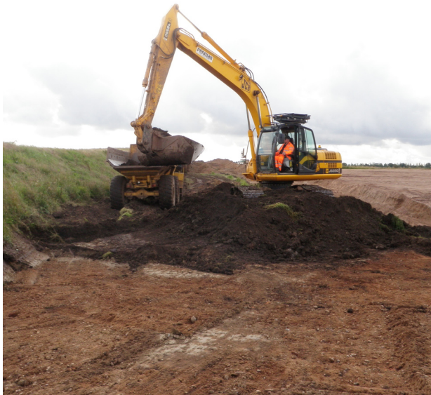
Illus 2 General view of topsoil stripping
