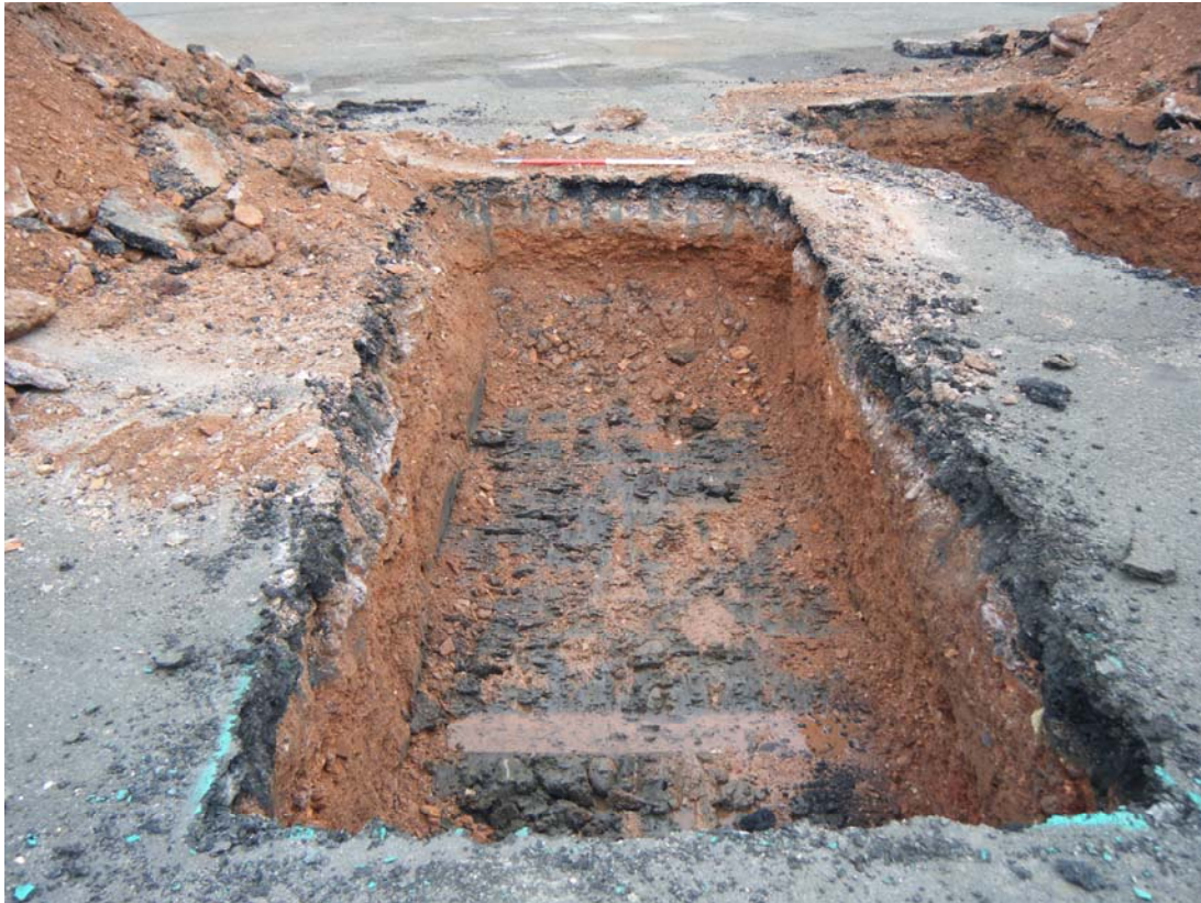
Illus 3 View of Trench 2
