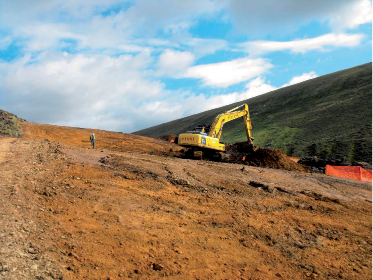
Illus 5 Monitoring topsoil stripping
