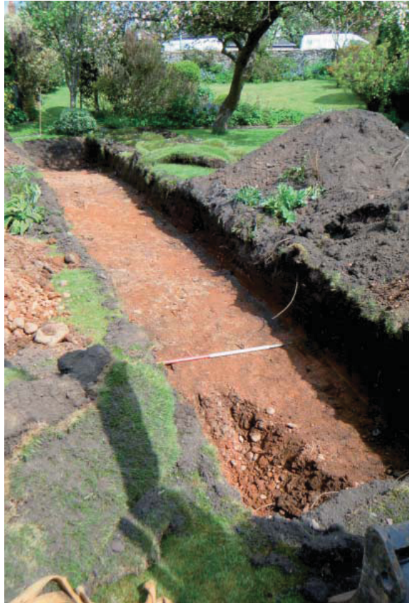
Illus 2 View of Tr. 1 from the south
