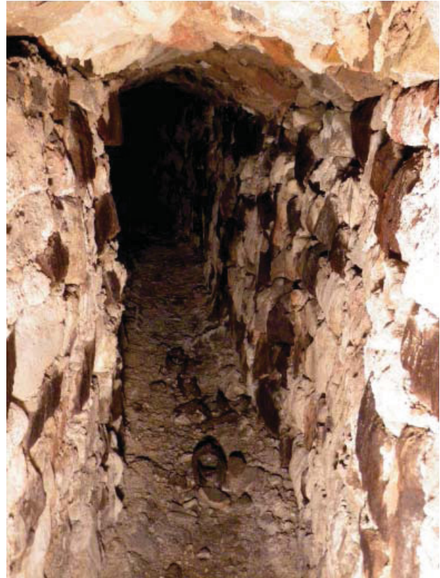
Illus 20 Culvert structure 6
