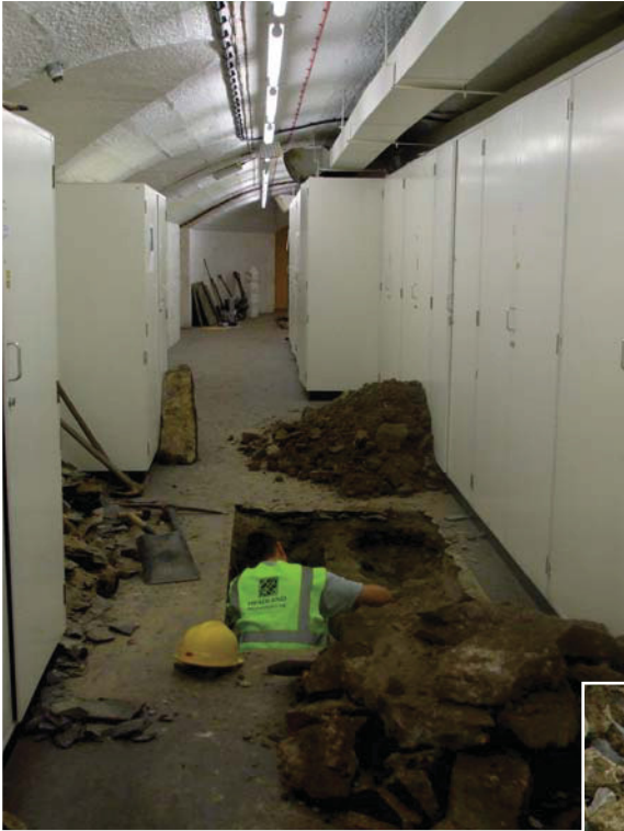
Illus 4 Working shot of test pit excavation
