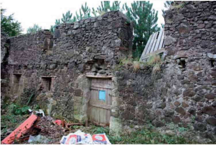
Illus 14 View of the west wall for Room C (from the north-east)
