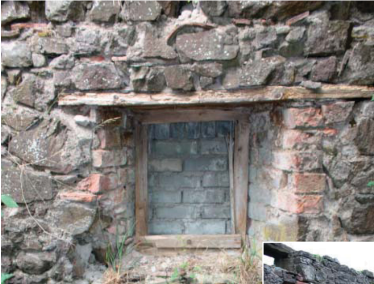
Illus 12 Internal view of the blocked door F01 (from the east)
