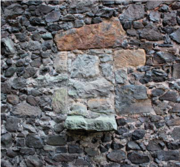
Illus 6 View of Window F19 (from the south)
