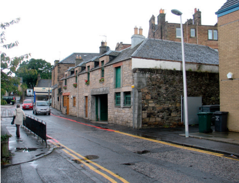
◀ Illus 7 Building A from Kirk Loan, showing boundary wall
