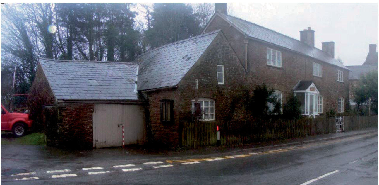
Illus 4 Plate 1 showing external view of the building
