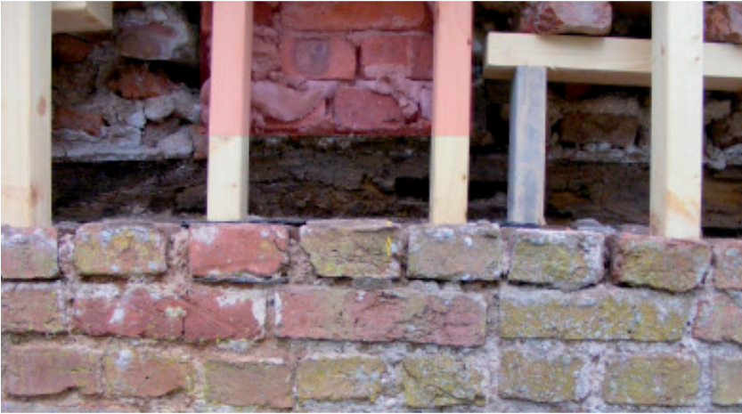
Illus 7 Area of modern brickwork (highlighted in red)
