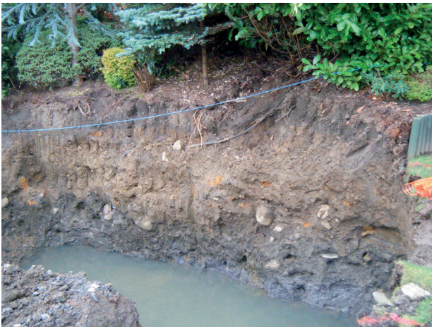
Illus 3 Deep excavation at NW end of the site, facing NW
