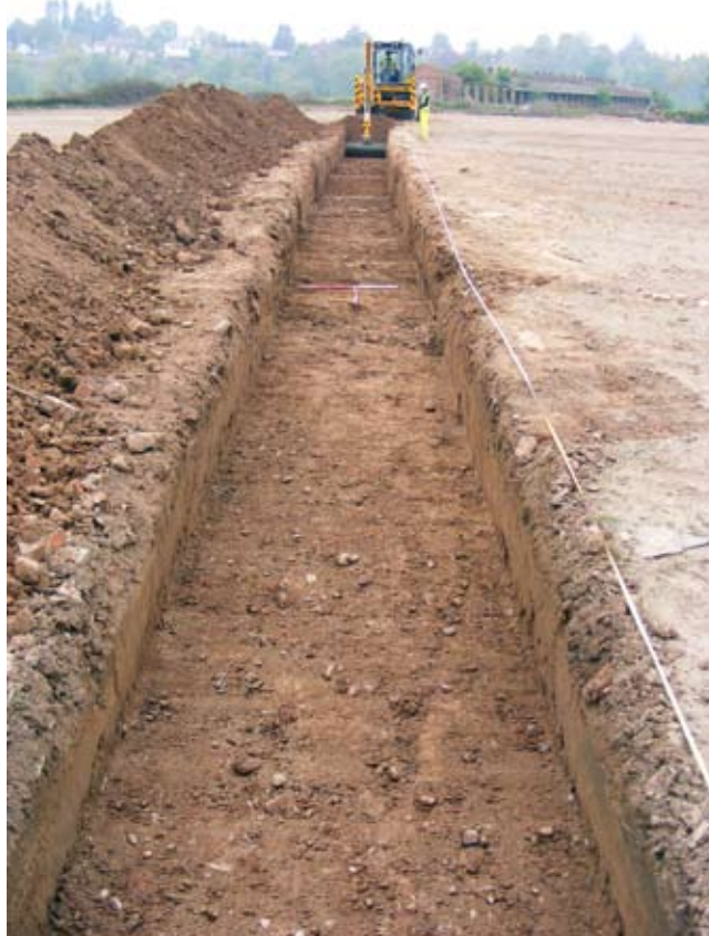
Illus 2 Excavation of Trench 1
