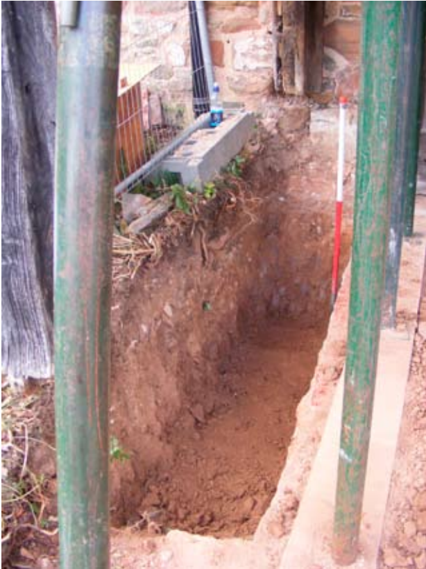
Illus 7 Trench 1 looking N
