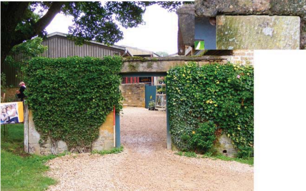
Carpark wall with insert illustrating the concrete lintel
