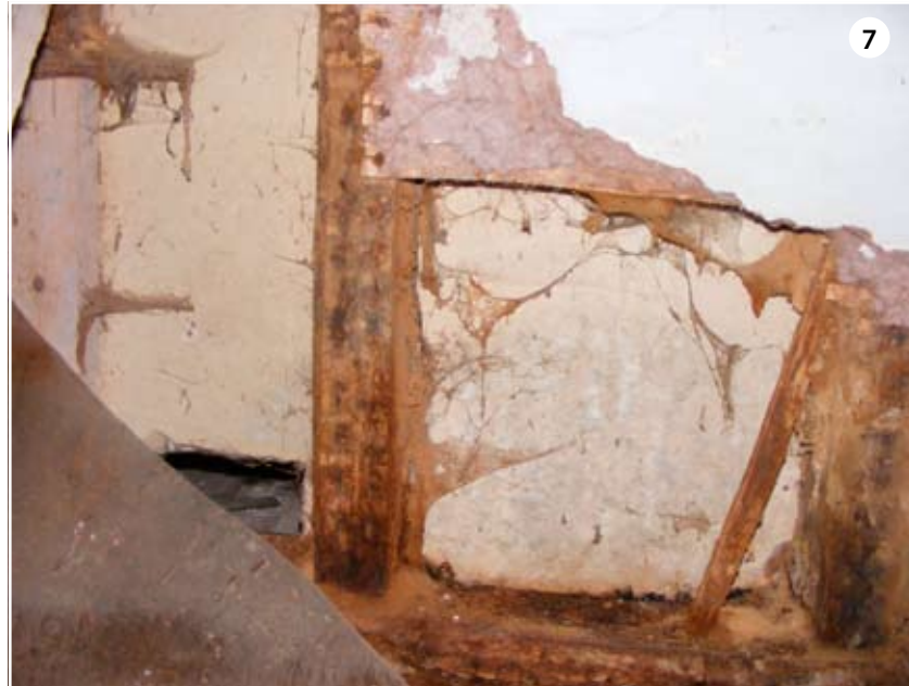
Detail showing construction of internal walls
