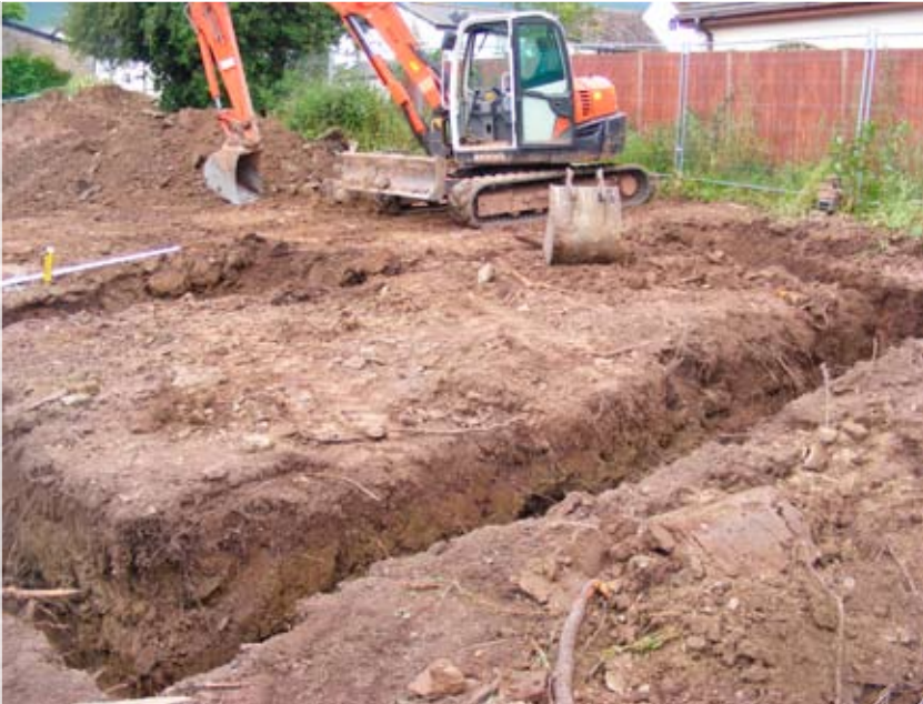
Excavated footings at the south of the site
