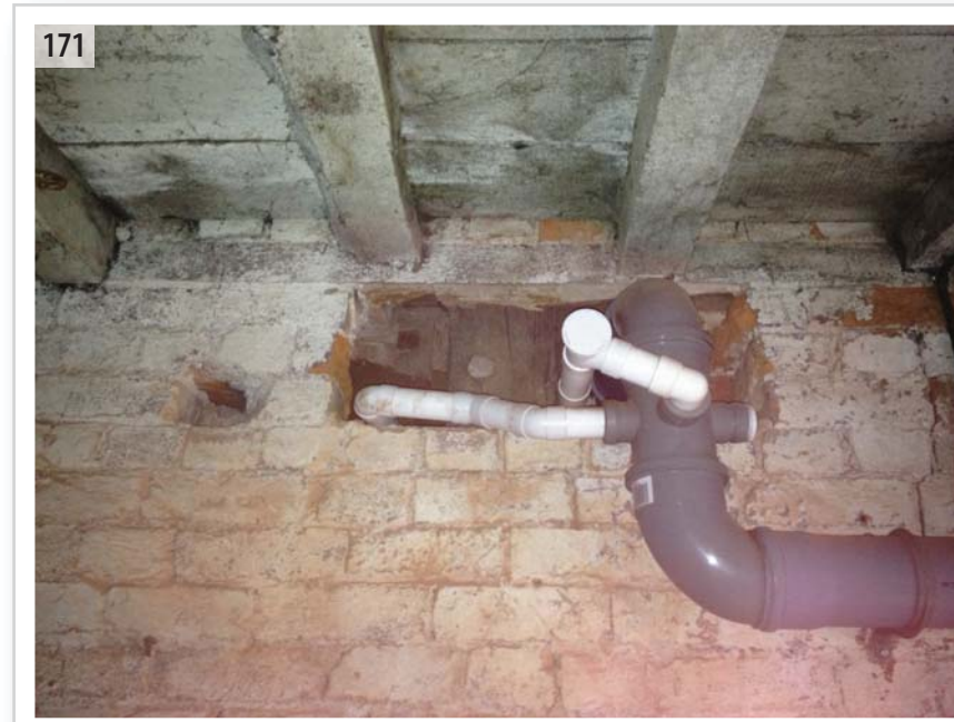
171 Internal view showing timber framing of abutting building, seen within modern hole cut for plumbing
