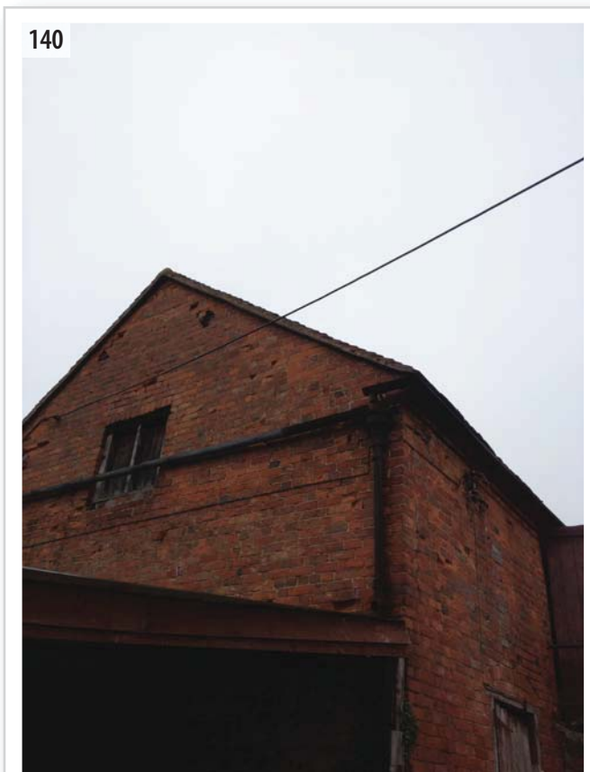
140 External view showing the gable end and change in coursing
