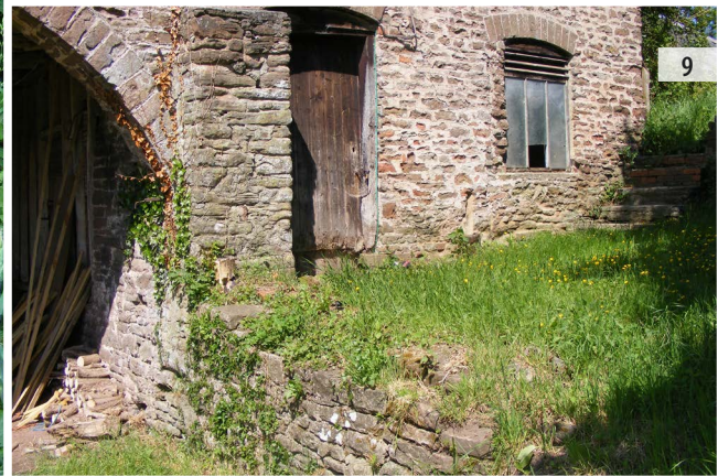
ILLUS 7 View of original mortar (135) ILLUS 8 Projecting masonry in the north wall of Building 1 (049) ILLUS 9 Buttress and retaining wall, indicating the location of a possible demolished building (128)
