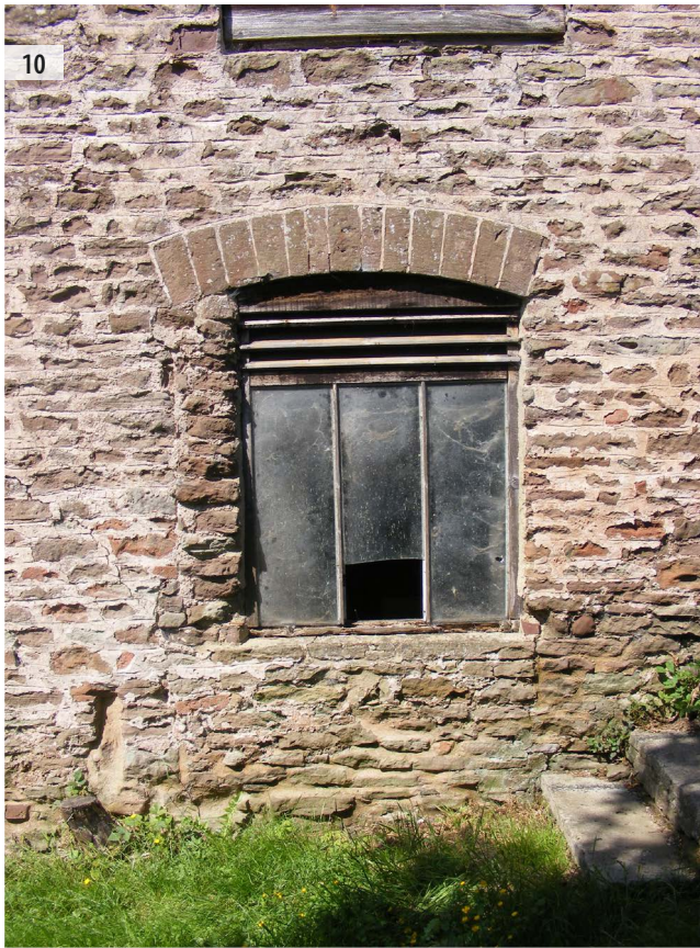
ILLUS 10 Later inserted window within an original doorway in Building 1 (124)
