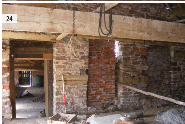
ILLUS 22 Inserted doorway, west elevation, Building 1, A2 (032) ILLUS 23 Projecting line of chimney breast A3, Building 1 (045) ILLUS 24 Blocked windows and converted window in southern elevation, Building 1, A3 (039)
