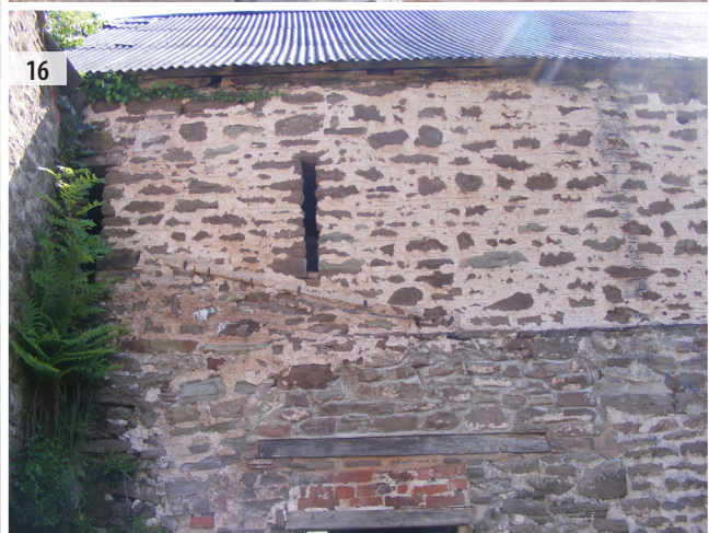
ILLUS 13 Building 1, west elevation Building 1 (106) ILLUS 14 Lancet window with later blocking and deliberate widening (105) ILLUS 15 Blocked door way, west elevation, Building 1 (106) ILLUS 16 Change in finishes indicating location of demolished building and later roof line, Building 1, west elevation (110)
