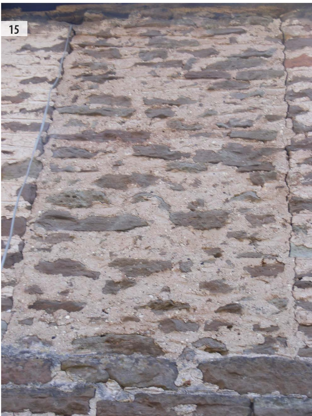
ILLUS 13 Building 1, west elevation Building 1 (106) ILLUS 14 Lancet window with later blocking and deliberate widening (105) ILLUS 15 Blocked door way, west elevation, Building 1 (106) ILLUS 16 Change in finishes indicating location of demolished building and later roof line, Building 1, west elevation (110)
