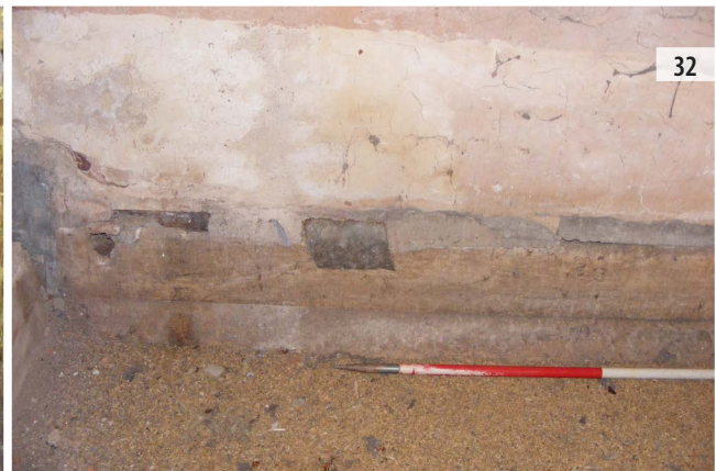
ILLUS 29 Internal roof details, Building 2 (034) ILLUS 30 Blocked doorway and inserted wall, Building 2, A1 (023) ILLUS 31 Interior of room B2 showing strap roller ILLUS 32 Angled and sealed skirting boards, Building 2, A4 (038)
