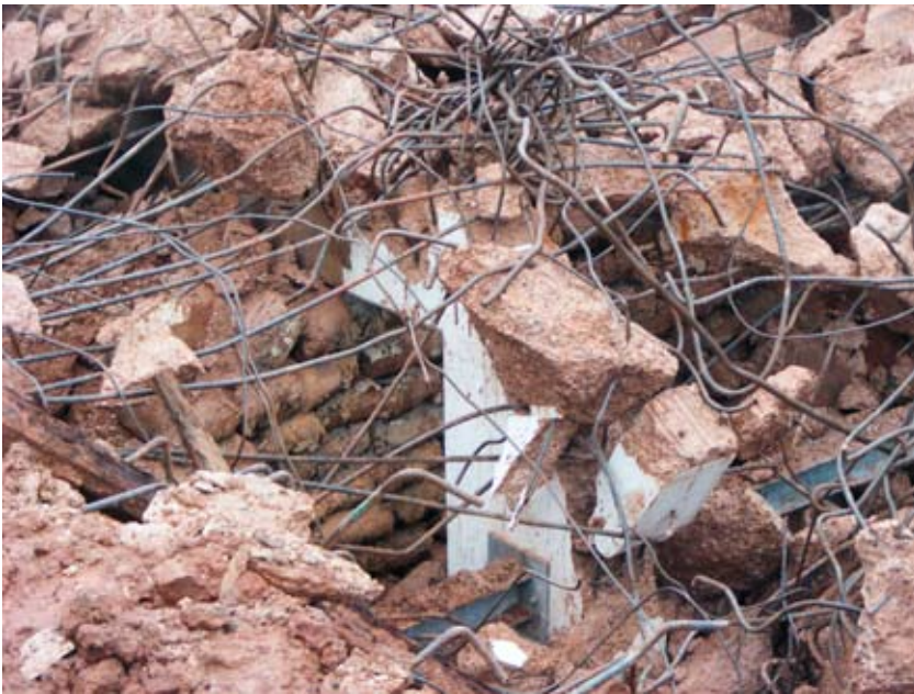
▲ Illus 8 Concrete bags in situ
