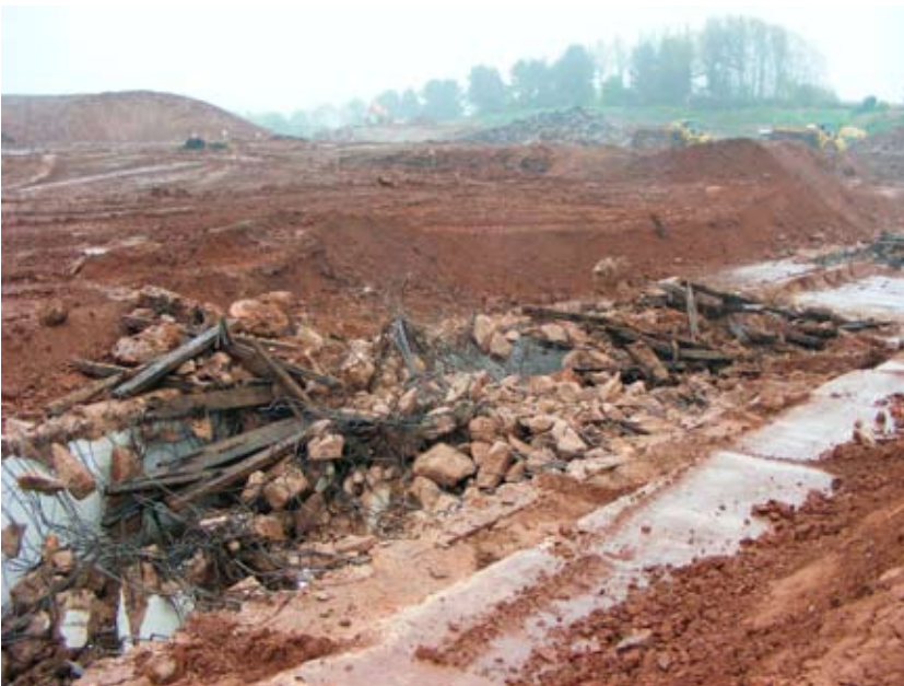
◀ Illus 6 Disturbed sleepers which formed the outer roof layer
