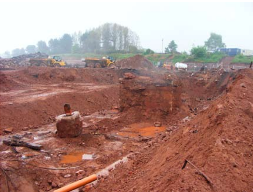
◀ Illus 7 Stairwell B – brick shaft to the surface
