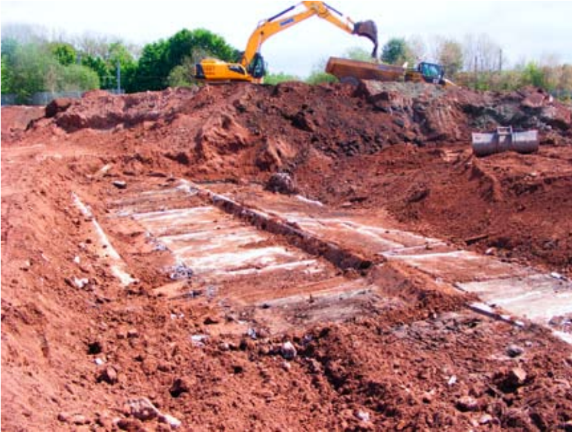
◀ Illus 5 Exposed roof with timber sleepers in situ
