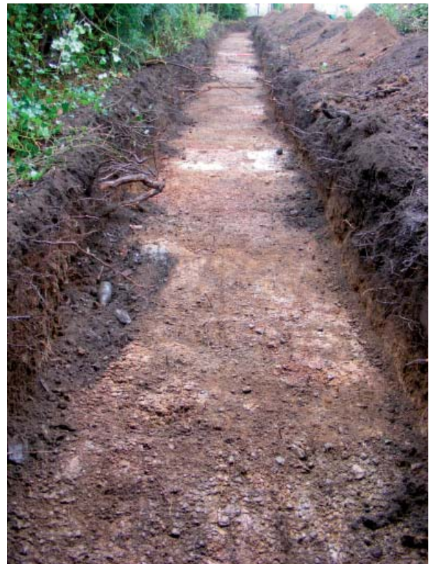
Illus 3 Trench 1 facing east
