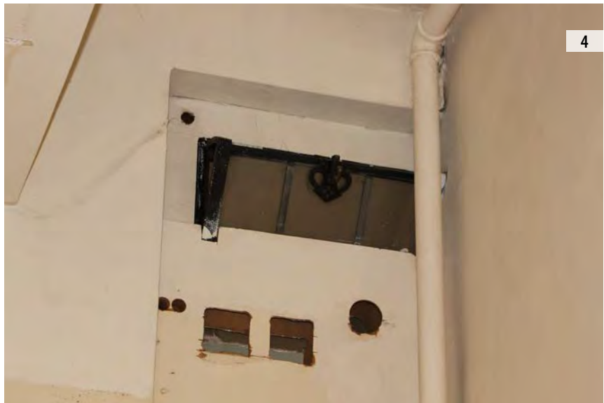
ILLUS 2 Example of window stay ILLUS 3 Example of window latch ILLUS 4 Hopper window ILLUS 5 Scroll end window stay
