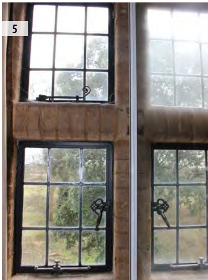
ILLUS 2 Example of window stay ILLUS 3 Example of window latch ILLUS 4 Hopper window ILLUS 5 Scroll end window stay
