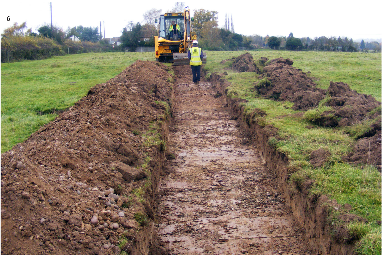
ILLUS 3 Trench 6, topographic section, facing W
