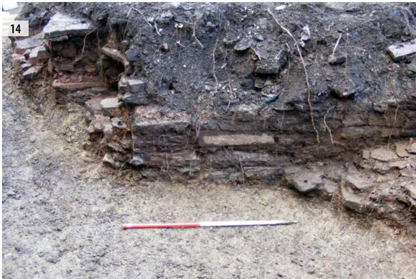
ILLUS 14 Wall foundation [016], looking west and east facing elevation of wall foundation [016]
