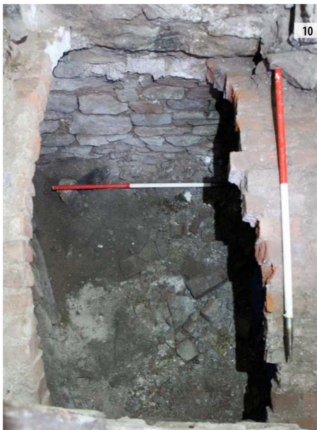
ILLUS 9 Trench 4, brick vaulting exposed below floor of extant Victorian building, facing north ILLUS 10 Trench 4, partially removed brick vaulting revealing void below prior to excavation, facing north ILLUS 11 Trench 4 facing east. View along the void beneath brick vaulting
