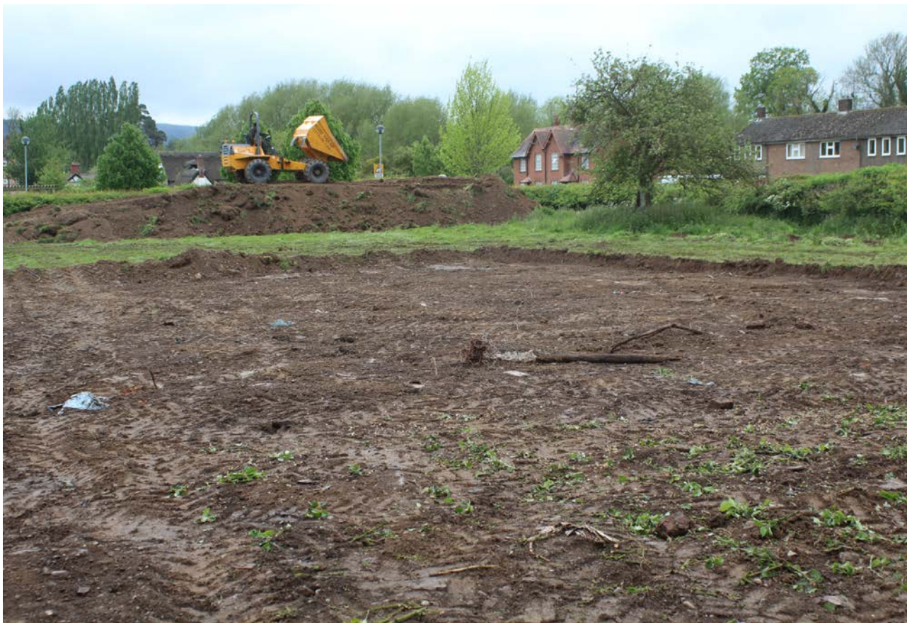
ILLUS 2 Stripped area facing SW
