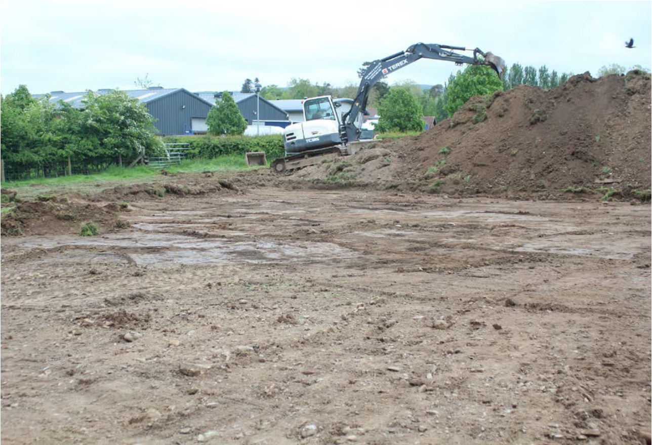
ILLUS 3 Stripped area facing SW
