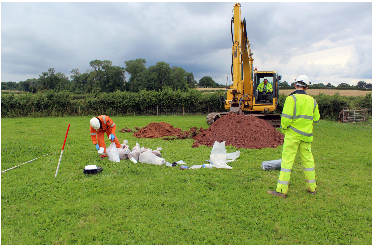
ILLUS2 General view work in progress, southern test pits, looking north-east
