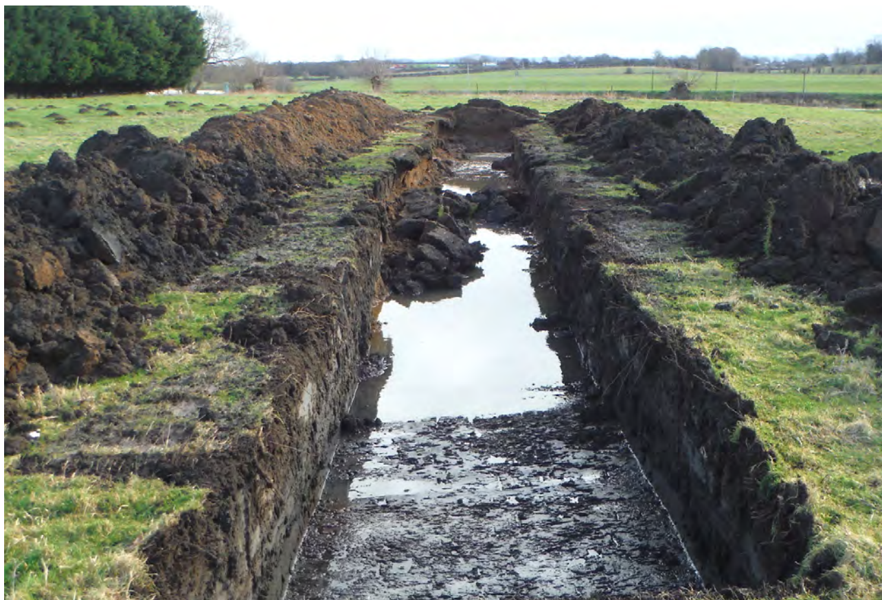
ILLUS 6 Trench 12 showing trench conditions to the east of the site
