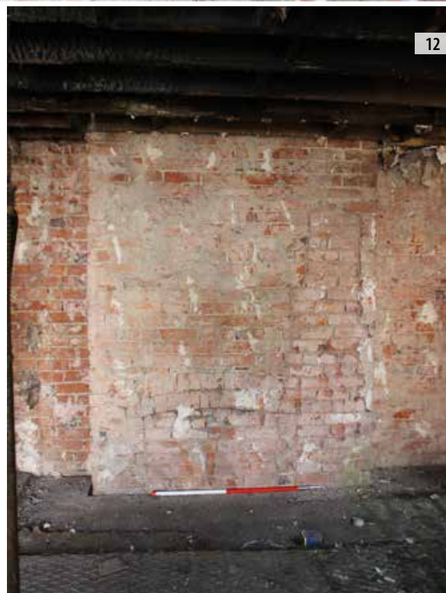
ILLUS 12 View of blocked fireplace, south wall of room 17
