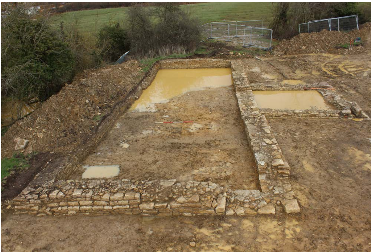
ILLUS 13 Building range [8241] showing facing, coursing internal and external elevations
