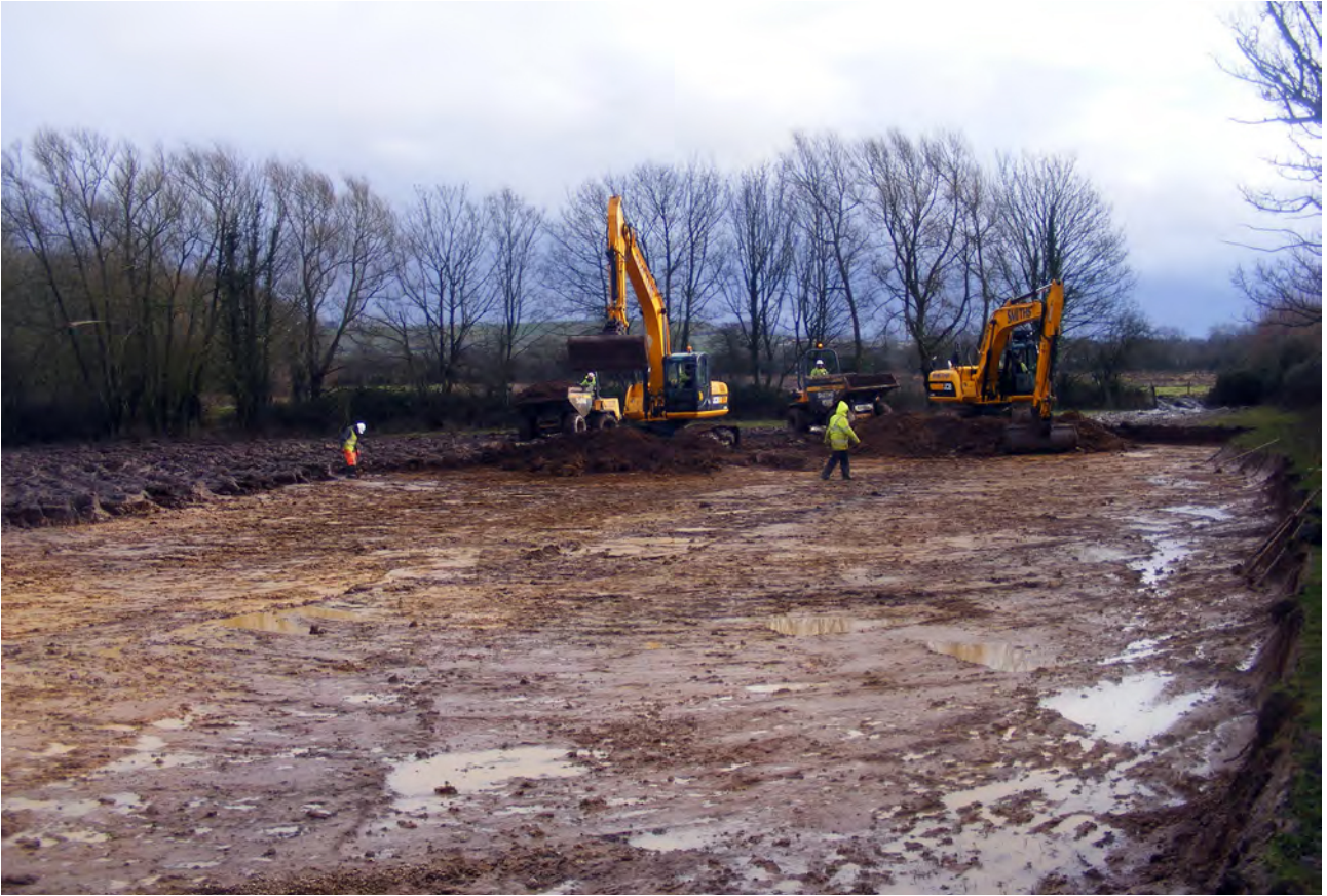
ILLUS 53 Working shot, Trench 4e, facing west
