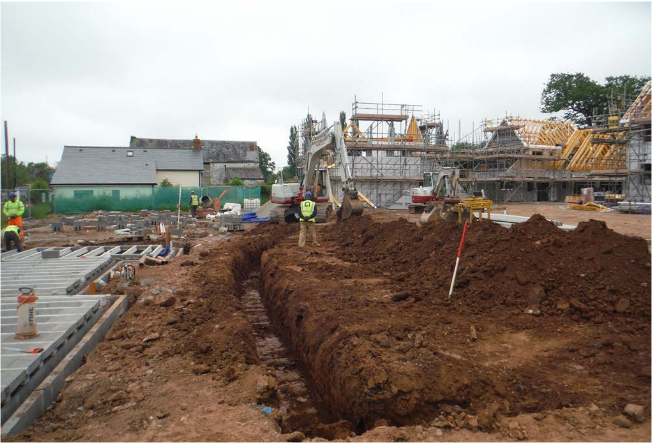
ILLUS 6 Trench 2 overview looking north-east
