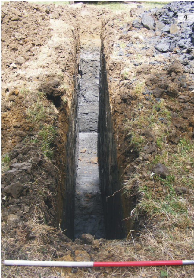
ILLUS 10 Storm drain in former field boundary ditch [012], Test Pit 2, looking south
