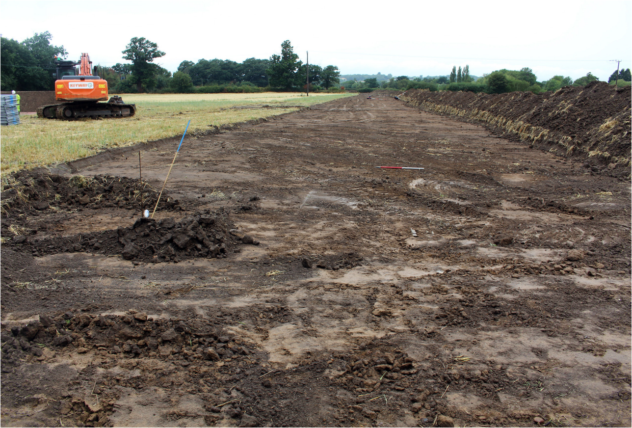
ILLUS 3 General view of pipeline easement, Field 1, looking west
