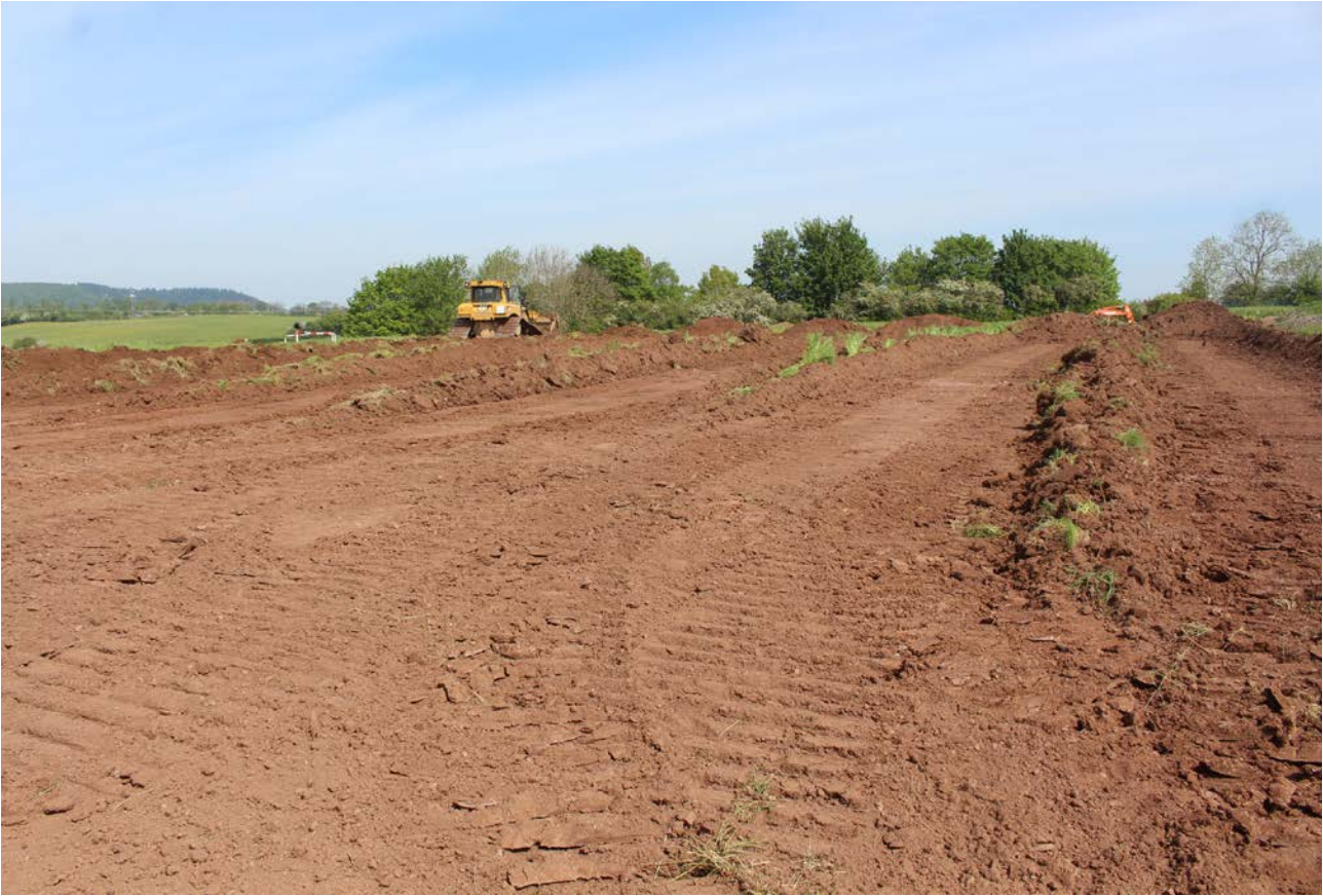
ILLUS 3 General view of bulldozer stripping reservoir area, looking north-east
