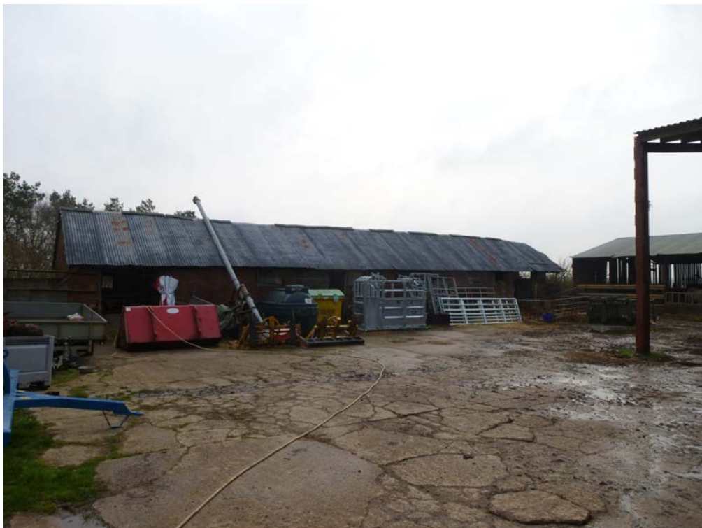
Image EDP 4: View of the farmyard looking east, showing the eastern range of outbuildings
