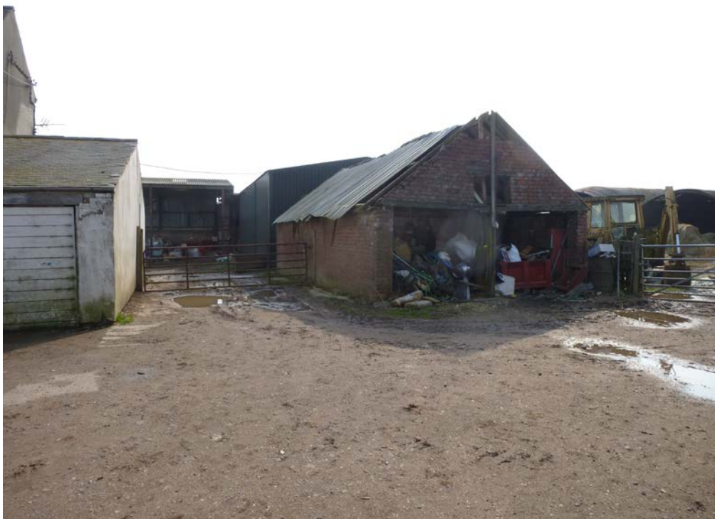
Image EDP 6: View of the remaining section of the west range of the farmyard, looking south with the farmhouse to the left
