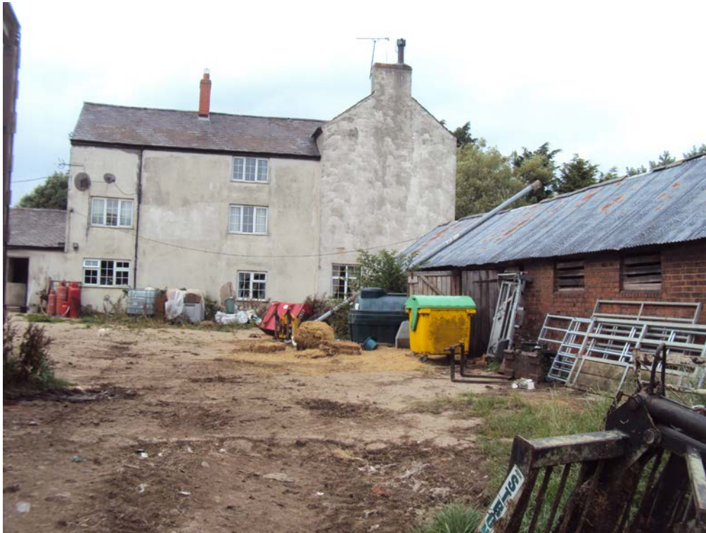
Image EDP 3: View of the farmyard from the south, showing the farmhouse and the eastern range of outbuildings
