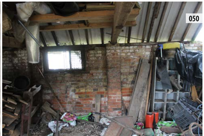
BUILDING 1 INTERNAL SPLL-HBR 051 SPLL-HBR 050
