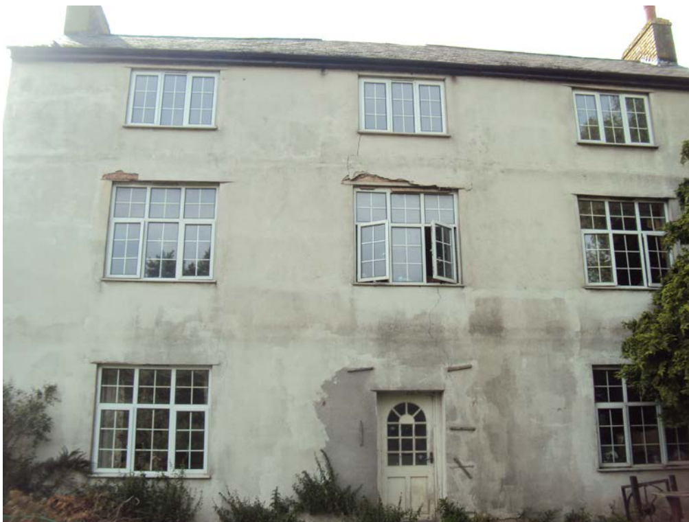
Image EDP 2: View of the farmhouse from the east
