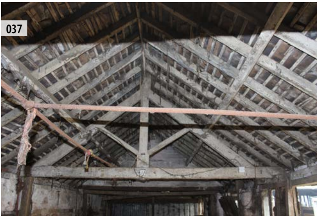
BUILDING 2 INTERNAL SPLL-HBR 037 SPLL-HBR 043
