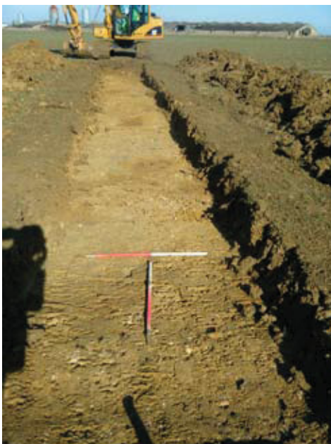
Photo 23 Trench 3 facing NW
