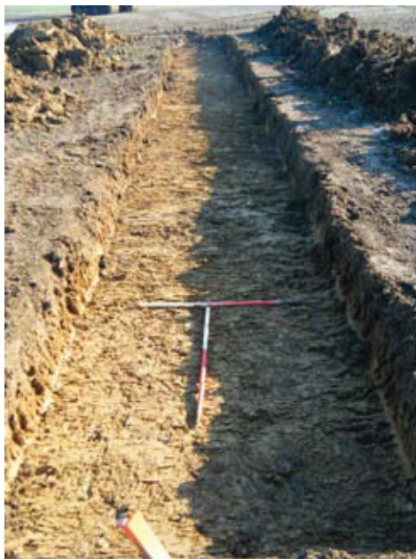
Photo 22 Trench 4 facing SW
