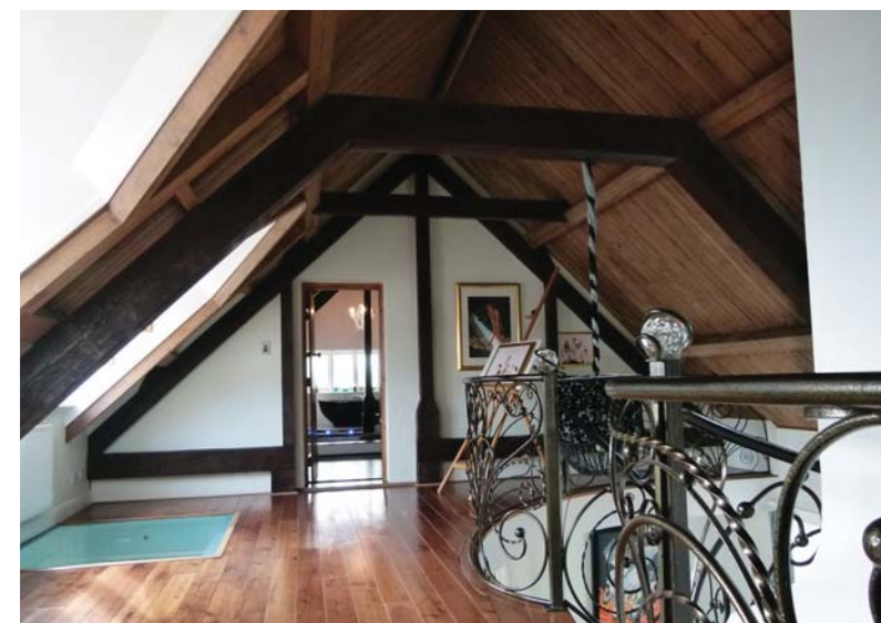
4 View of original roof beams and modern redevelopment from the north-west
