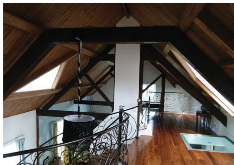
3 View of original roof beams and modern redevelopment from the south-east
