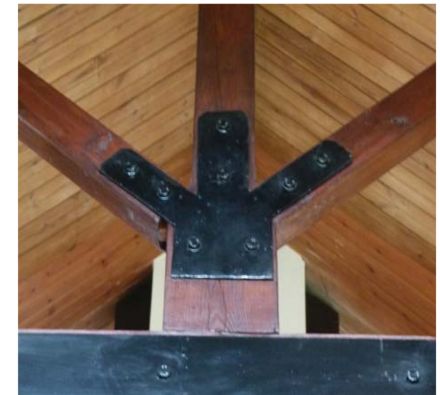
5 Modern metal joint added to existing roof trusses, looking north-west
