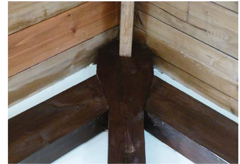
6 Detail of original roof trusses joint and modern roof, looking south-east
