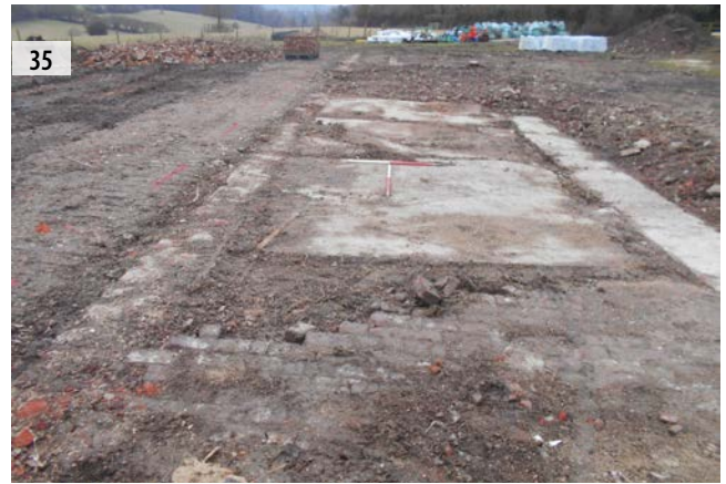
ILLUS 33 SMS Area 1, facing south ILLUS 34 Sample section Area 1, west facing section ILLUS 35 SMS Area 2, facing west, in situ 19th century floor in foreground of image
