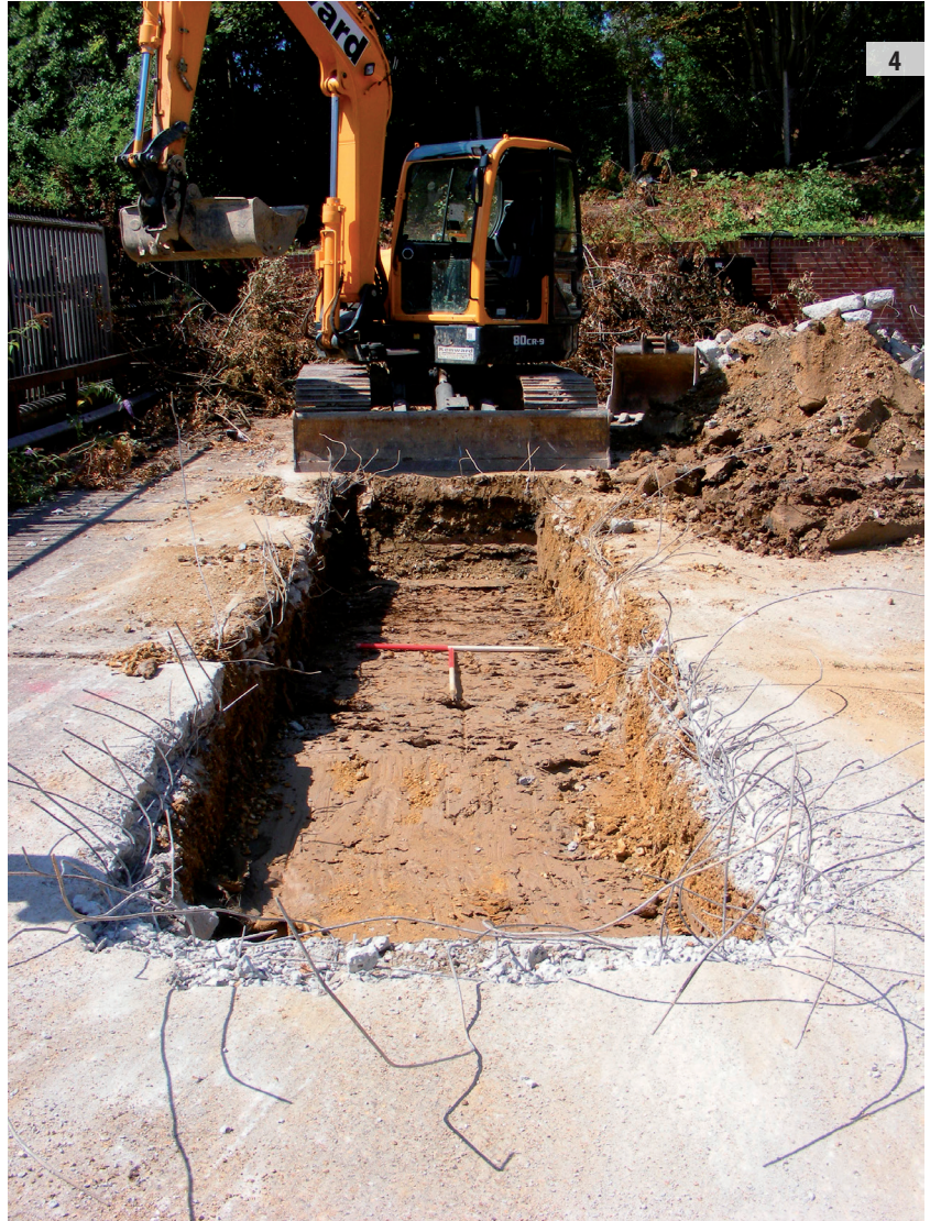
ILLUS 4 Trench 2, looking SW
