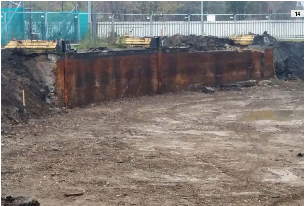
ILLUS 14 Area 4 overview, facing north-east
