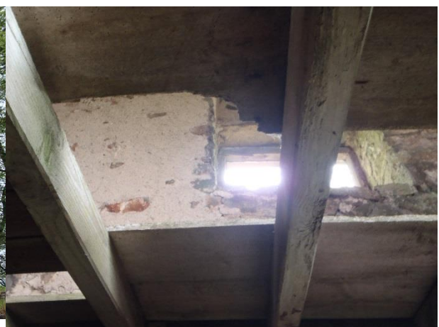
Plate 32: view into 6A through hole in ceiling of Room 6
