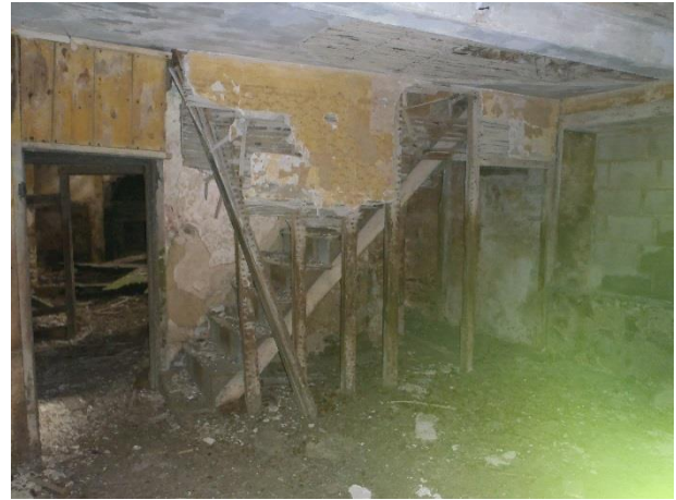
Plate 16: stud wall and stairs in Room 3 with doorways into Room 5
