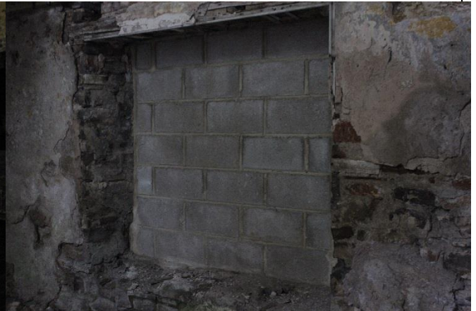
Plate 22: blocked window in south wall of Room 5
