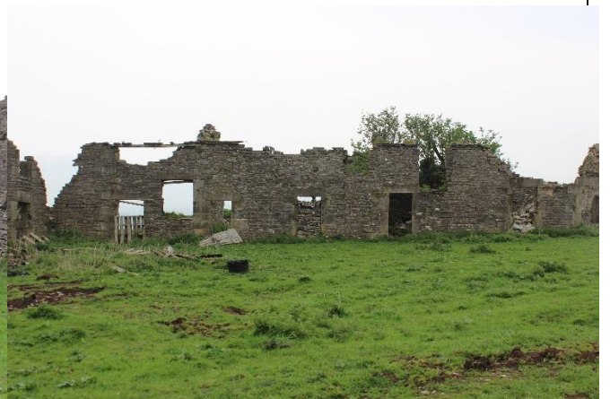
Plate 38: former large opening in west facing elevation of Outbuilding B
