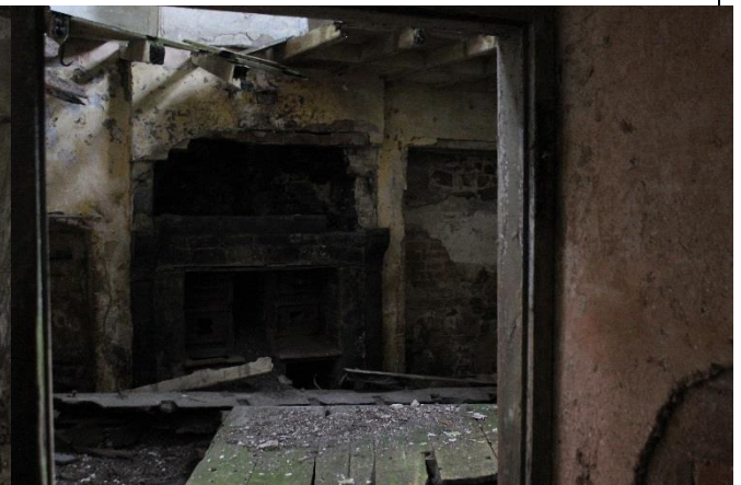
Plate 20: large range in kitchen (Room 5)
