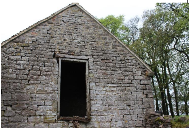
Plate 31: stone arch over upper floor doorway into 6A
