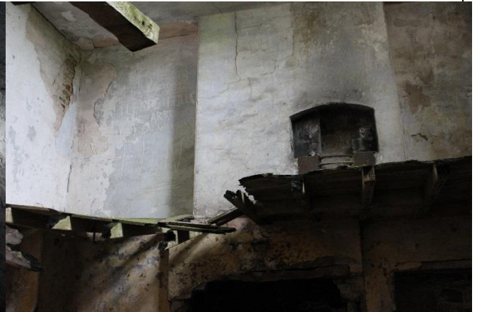
Plate 28: chimney breast and fireplace in Room 11 viewed from Room 5
