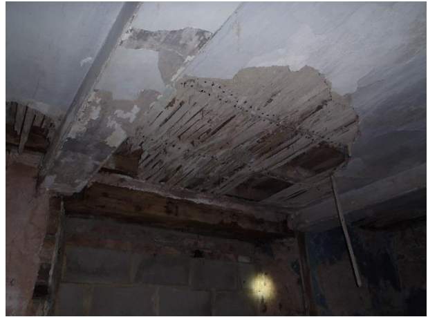
Plate 10: Ceiling and beams in Room 1
