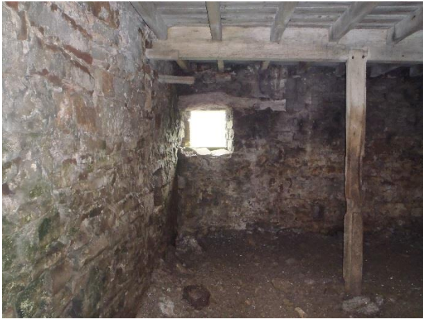
Plate 33: view of beam and supporting post in Room 6
