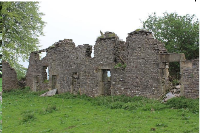
Plate 36: Outbuilding B from southwest
