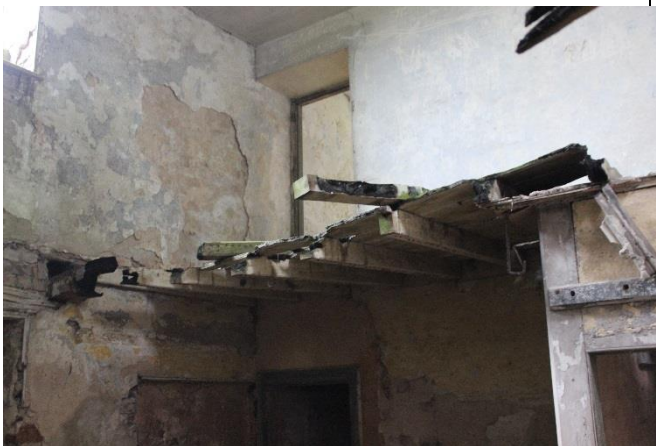
Plate 29: doorway from Room 11 into Room 10 viewed from Room 5
