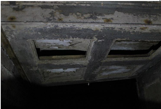
Plate 17: detail of door casing between Room 3 and Room 1
