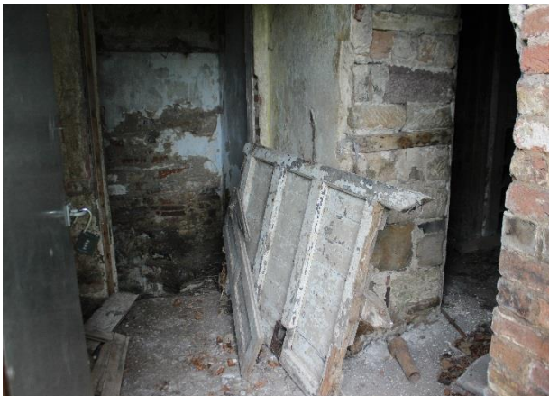
Plate 13: entry lobby with plank and batten door
