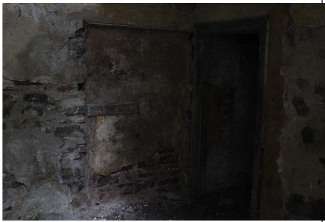
Plate 23: Blocked doorway in south wall of Room 5
