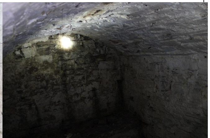
Plate 26: basement viewed from stairs
