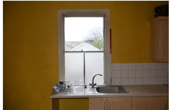
ILLUS 15: Original window with etched glass
