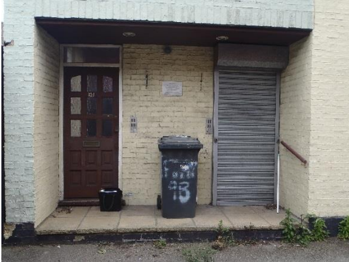
ILLUS 8: Later inserted doorways set in recessed opening
