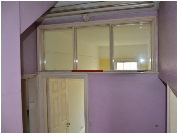
ILLUS 14: Additional window to provide illumination to the lobby area
