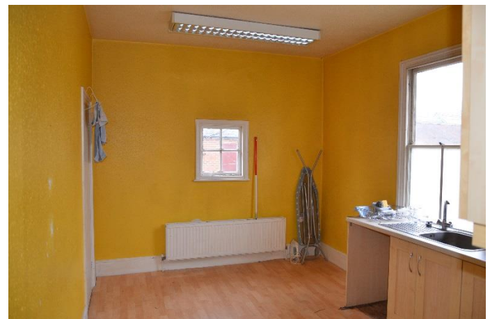
ILLUS 16: Single side opening casement window set in single skin wall
