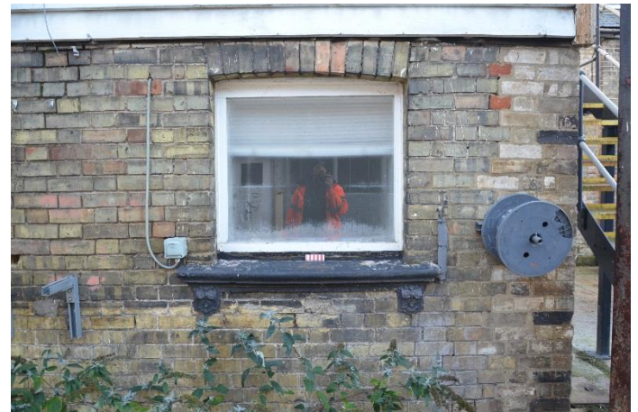
ILLUS 22: Detail showing cast iron window sill and decorative brackets
