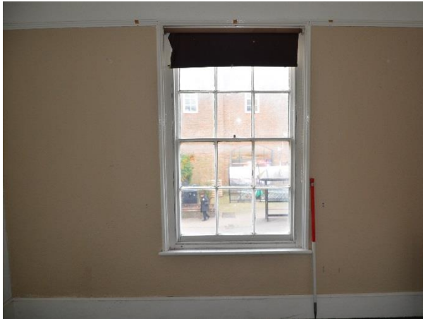
ILLUS 13: Original 12 pane sash window and skirting
