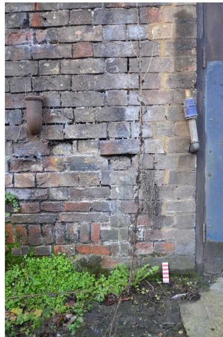
ILLUS 26: Coursing of handmade bricks and construction break between buildings G and H
