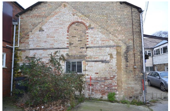
ILLUS 23: Blocked doorway and window opening with building scar
