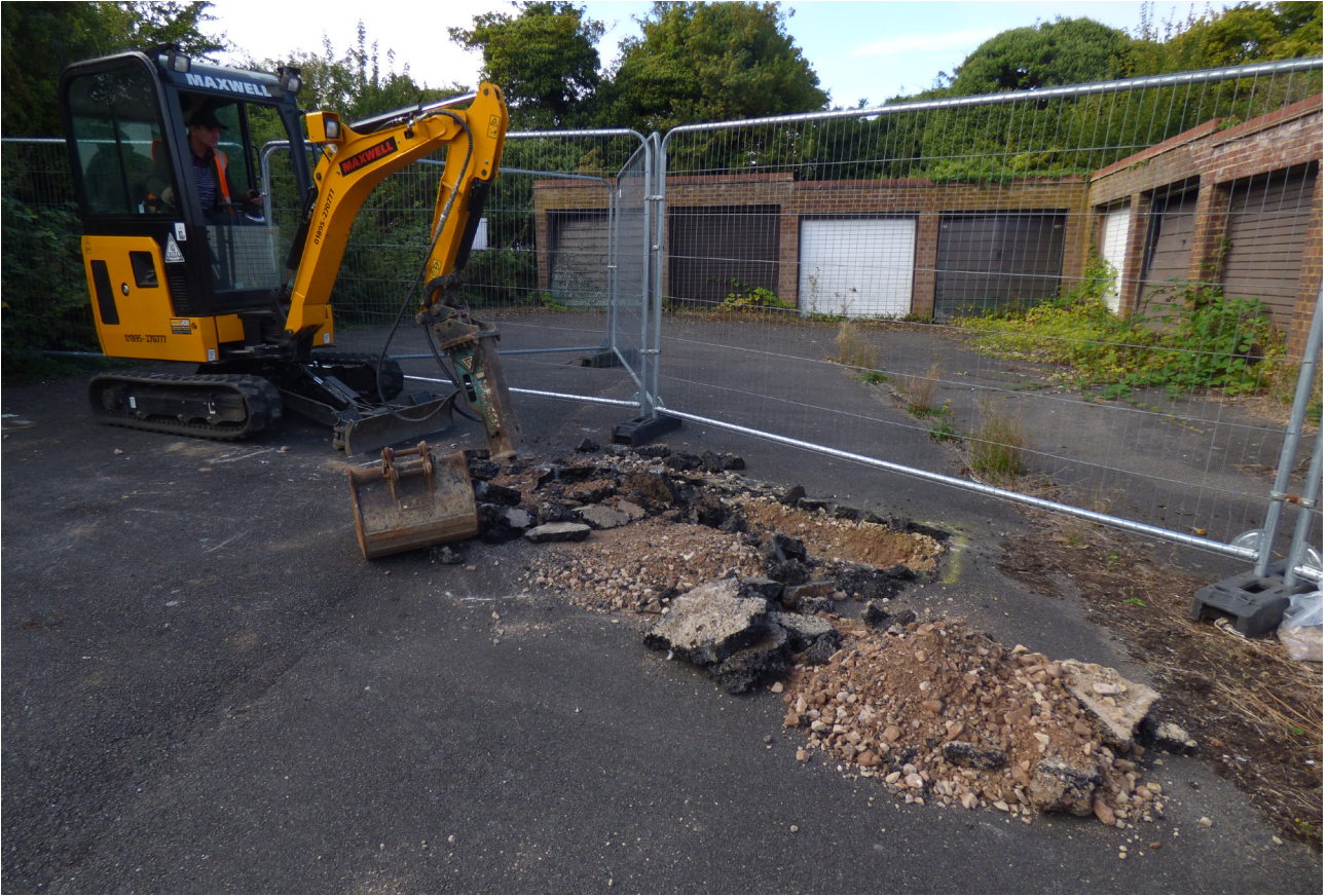
ILLUS 2 Trial Pit 4 during excavation, looking south
