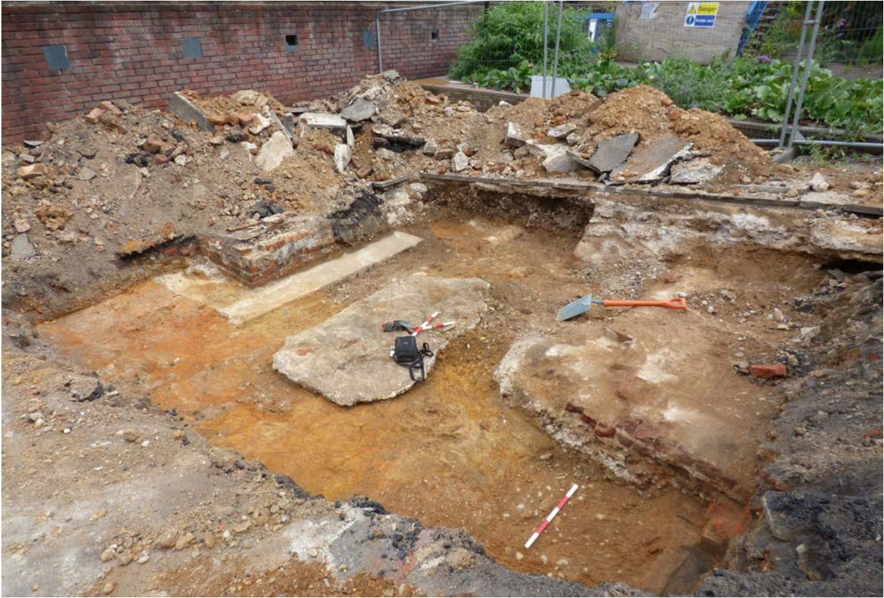
ILLUS 3 North-east facing working shot of site
