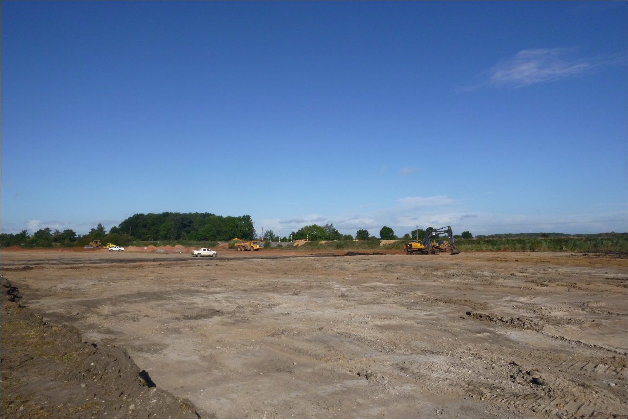
ILLUS 3 Field 5 (west), looking north
