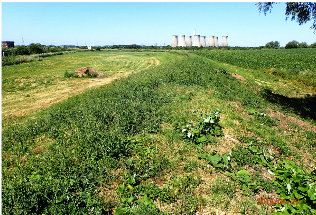
ILLUS 3 Existing flood defence embankment (south), looking west
