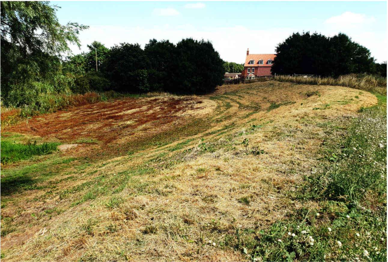
ILLUS 4 Existing flood defence embankment (south), looking east
