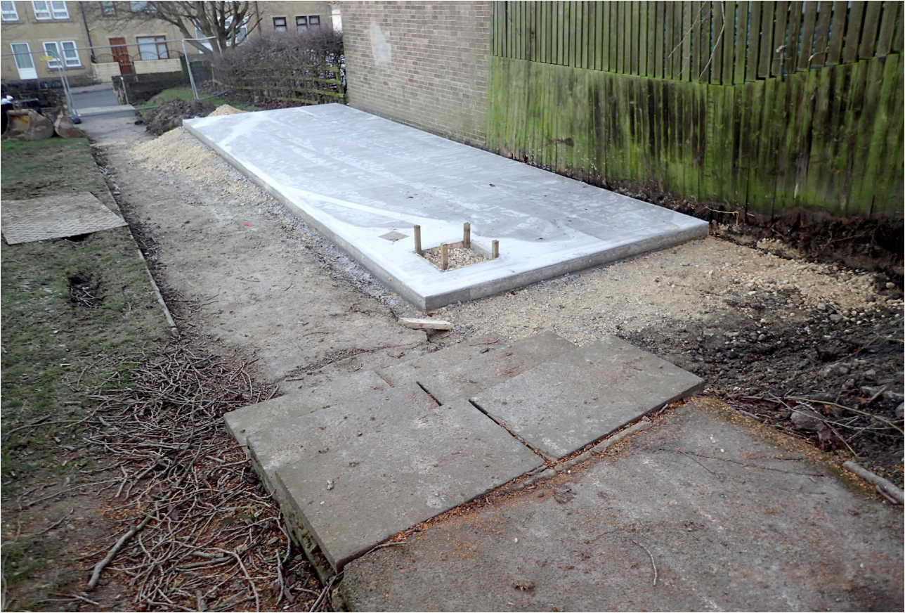
ILLUS 3 Concrete boiler base built prior to attending archaeologist
