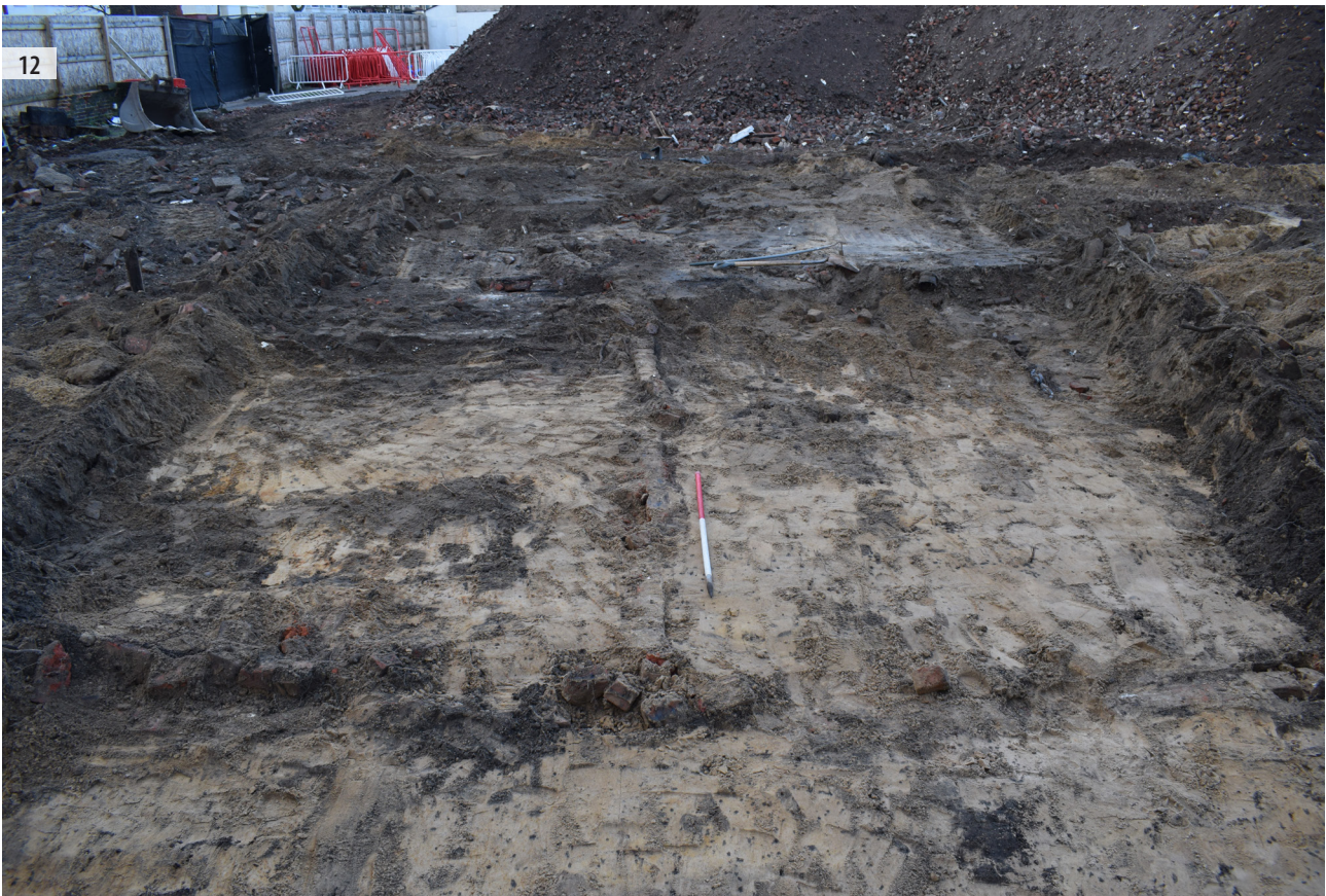
ILLUS 11 View of Trench 1 looking east. Context 3 is in the foreground ILLUS 12 View of Trench 2 looking west. Context 4 is in the foreground
